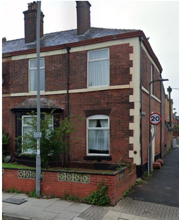
Figure 1: Front Elevation (Google Street View dated Aug 2023, Accessed May 2025)
