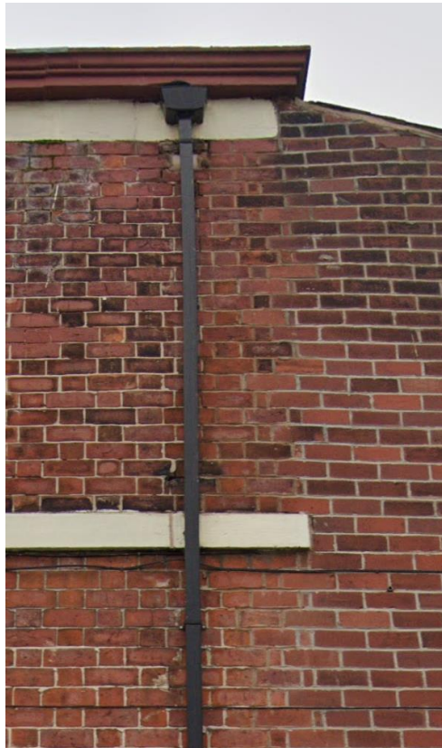
Figure 5: Features of the property: end of original form (Google Street View, dated Aug 2023, Accessed 22/05/2025)
