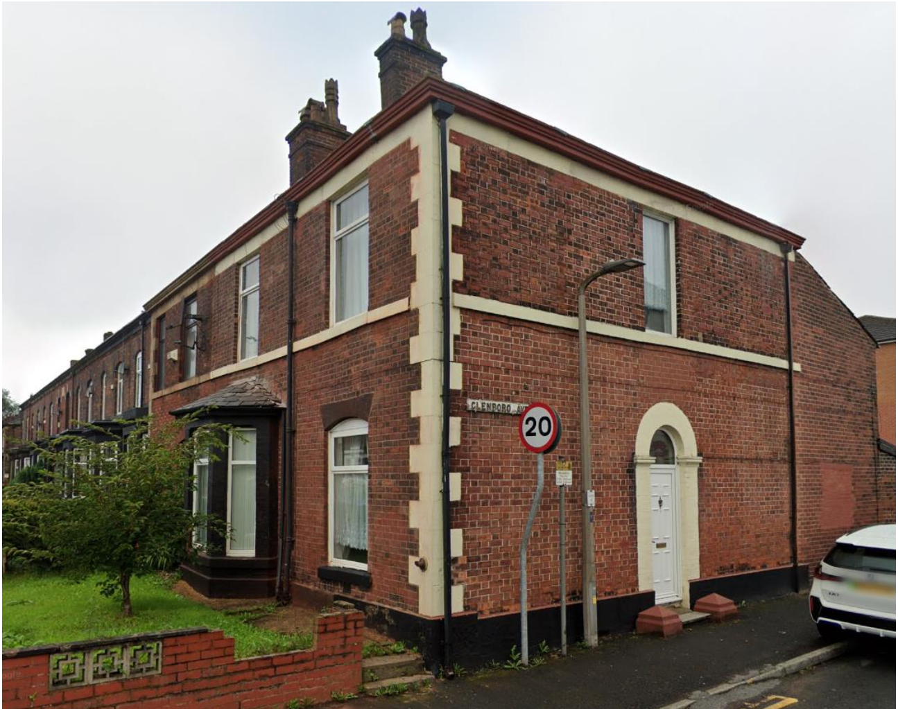
Figure 1: Front and Side Elevation and Entrance of 240 Bolton Road, Bury- Google Street View, Dated Aug 2023, Accessed May 2025
