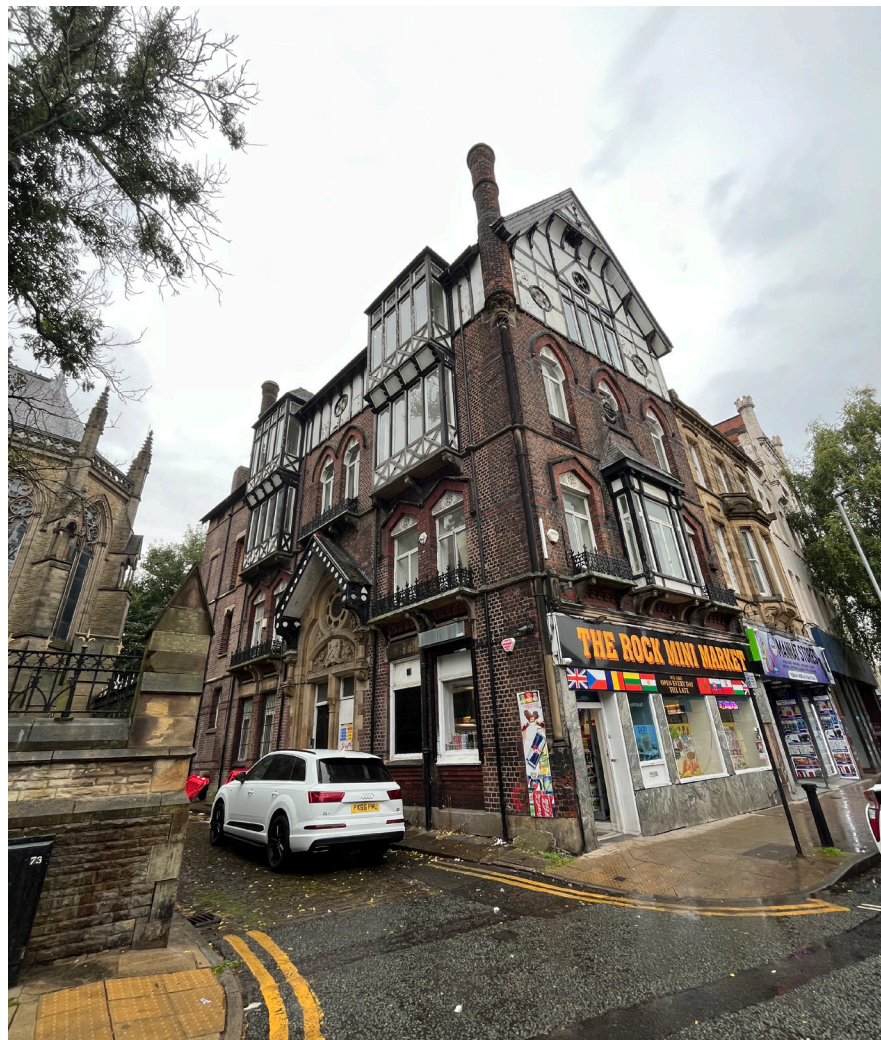
Image: Exterior of Union Club Buildings, 1 The Rock, Bury showing the two primary elevations.
