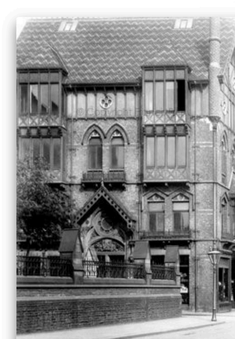
Image: 1895 view of Union Buildings showing original roof covering (no longer present).
