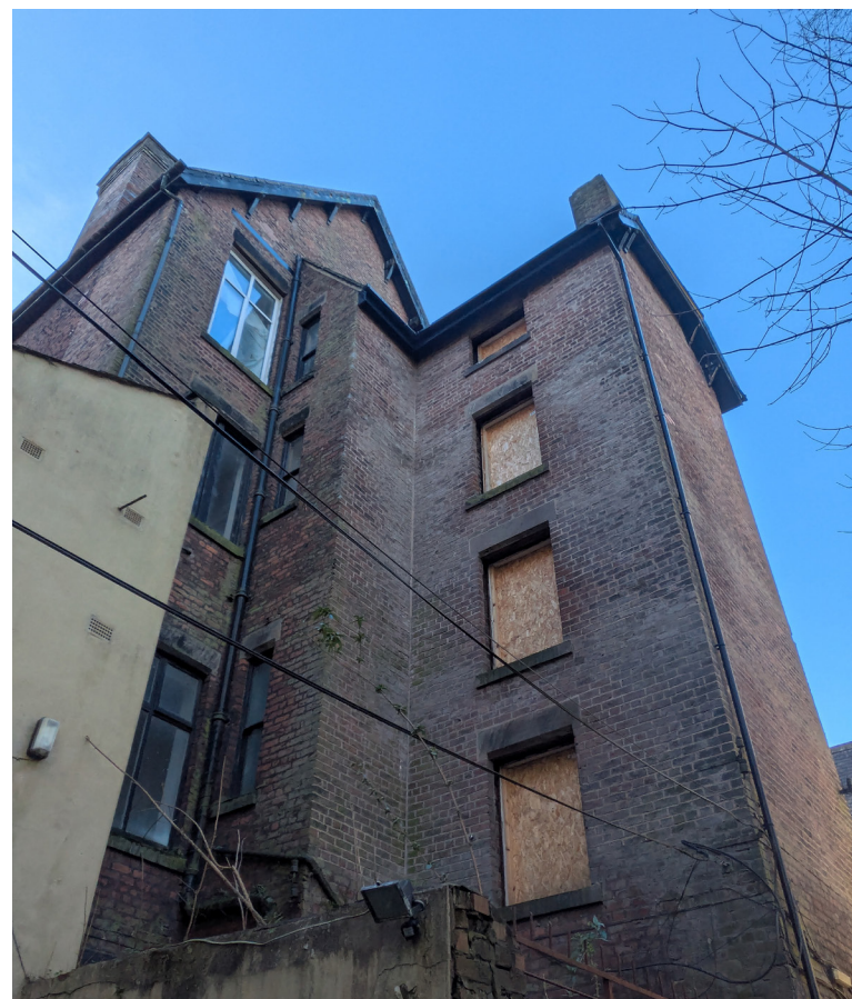
Image: Photograph showing the rear elevation of the building.
