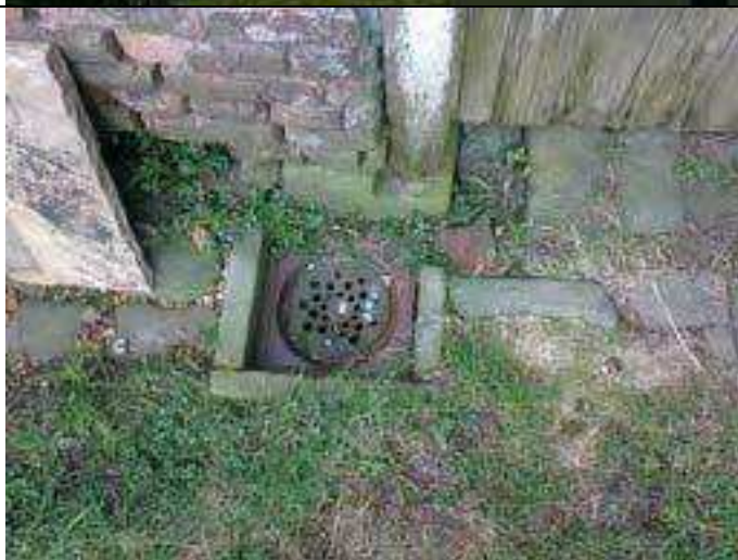
Photograph 8: Drain for the building to the north west of the site.
