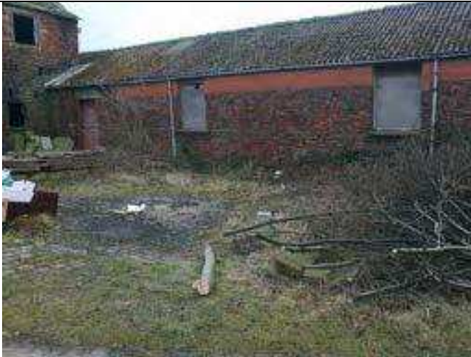
Photograph 4 (facing N): Original farm buildings to the north of the site.
