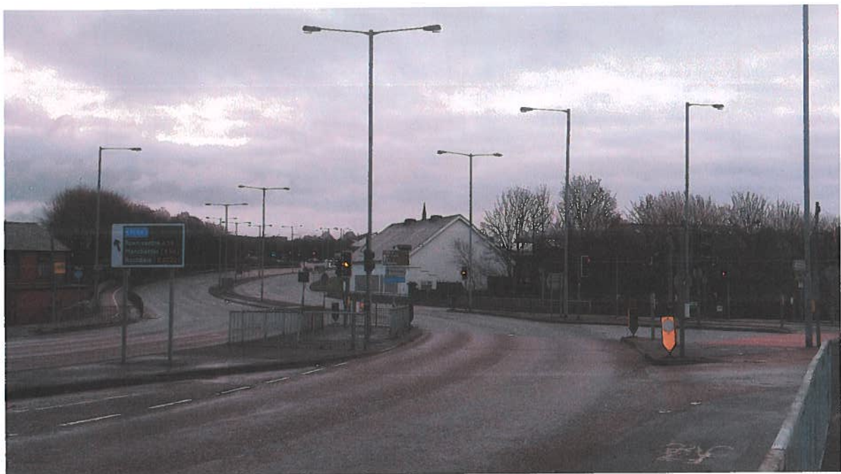
Pic 2 View on eastbound approach (taken from Crostons Rd).
