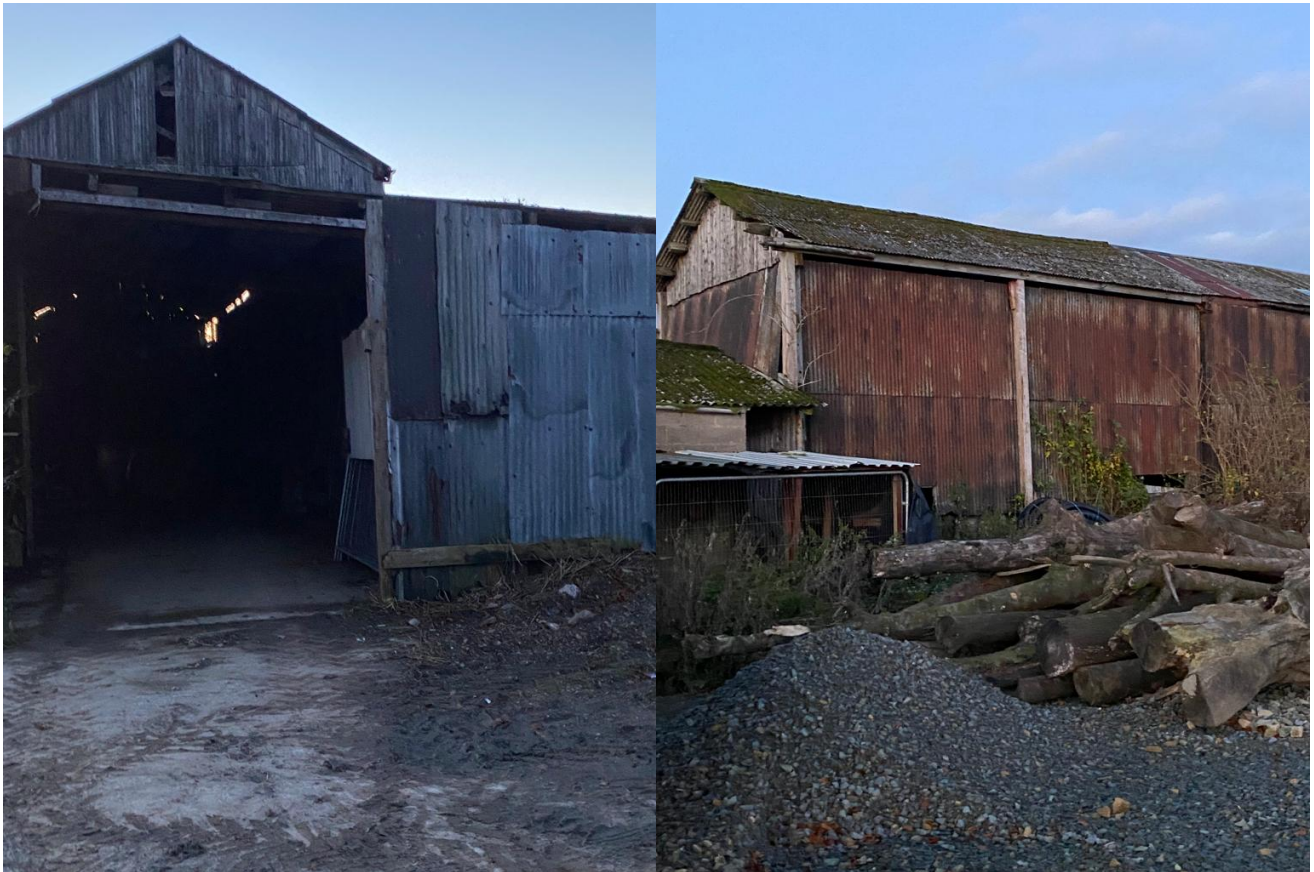
Shed to be lost is of simple timber framed construction with steel and timber cladding
