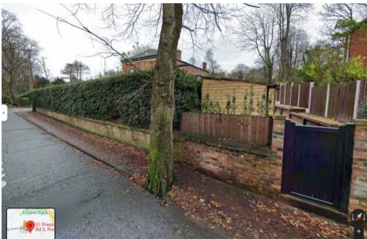
View on St Ann's Road towards the junction with Prestwich Park Road South, No 51 to the right (indicating previously closed vehicular entrance)
