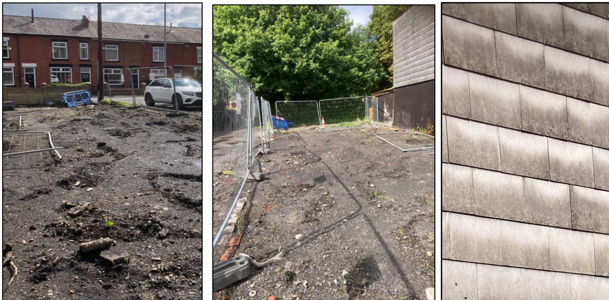
Images of former Ainsworth Garage site. View looking east (lhs,) view looking west (rhs) and close up of fibre cement tiles, sealed with no suitable gaps for use by bats
