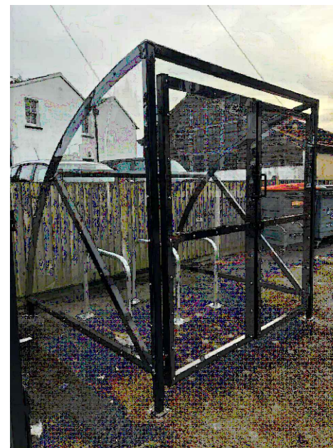
GALVANISED STEEL FRAMED CYCLE STORAGE SHELTER, FOR 8 CYCLES, 4100mm LONG x 2200mm DEEP/WIDE x 2200mm HIGH, WITH ANTI-VANDAL, UV STABLE POLYCARBONATE ROOF AND SIDE PANELS ALONG WITH SECURE LOCKABLE DOUBLE GATES. PROVIDE 4no SHEFFIELD STANDS, FIXED TO TO HARD STANDING. WITH 900MM GAP BETWEEN SHEFFIELD STANDS AND 550MM BETWEEN THE STANDS AND SIDE FRAME OF SHELTER, AS DIMENSIONED
