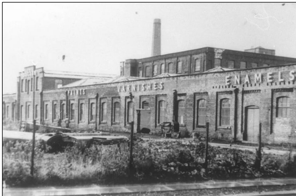
Figure 6 – Site photograph taken from the 'Warth Mills Project' website showing the main mill building during the time that the site was used as a paint and varnishes factory. Photograph is believed to be taken from Warth Road to the north east of site.
