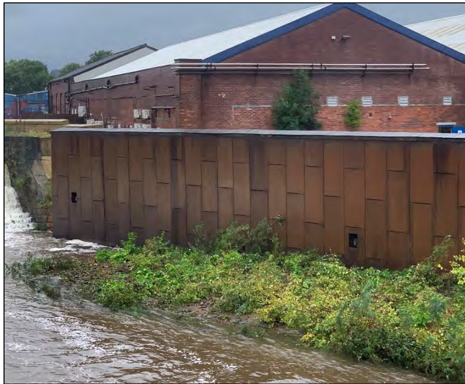
Figure 14 – Photo taken from off site to the south east looking north west back onto site at the recently installed retaining wall. 2 No. outfalls can be seen, neither of which appear to have any water flowing from them. Photo taken 20 th September 2023.
