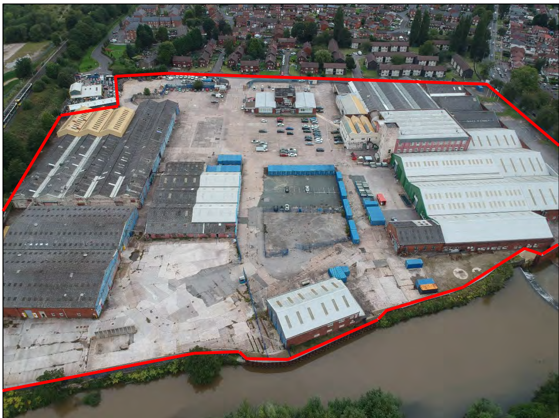
Figure 1 - Aerial image of the site dated August 2023. The approximate site boundary is highlighted in red.
