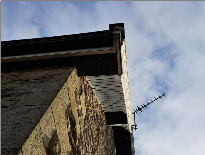
Photograph 7 showing the uPVC soffits
