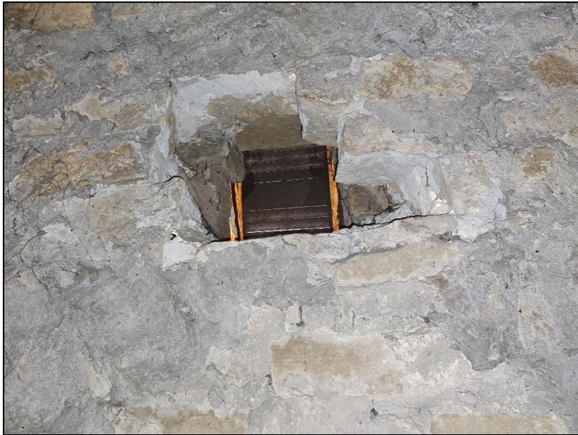
Photograph 17 showing one of the louvre windows
