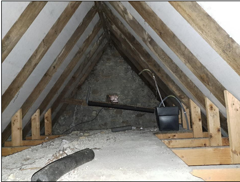
Photograph 15 showing roof void
