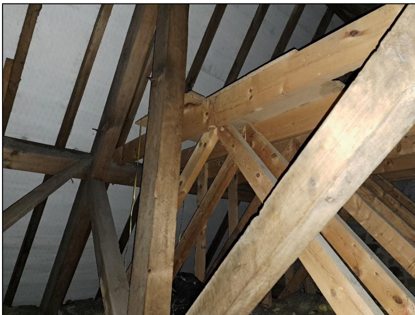
Photograph 16 showing the timber and the lining
