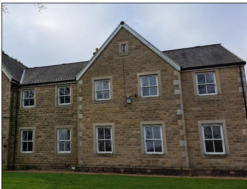
Photograph 1 showing the eastern elevation
