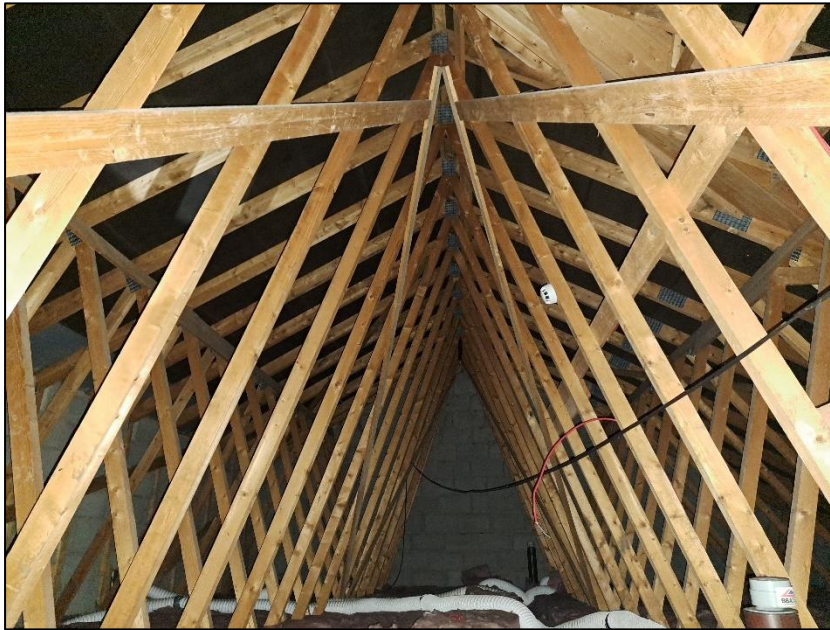
Photograph 9 showing the roof void
