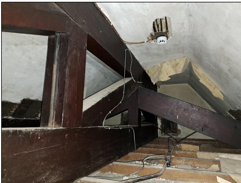
Photograph 14 showing one of the original roof voids
