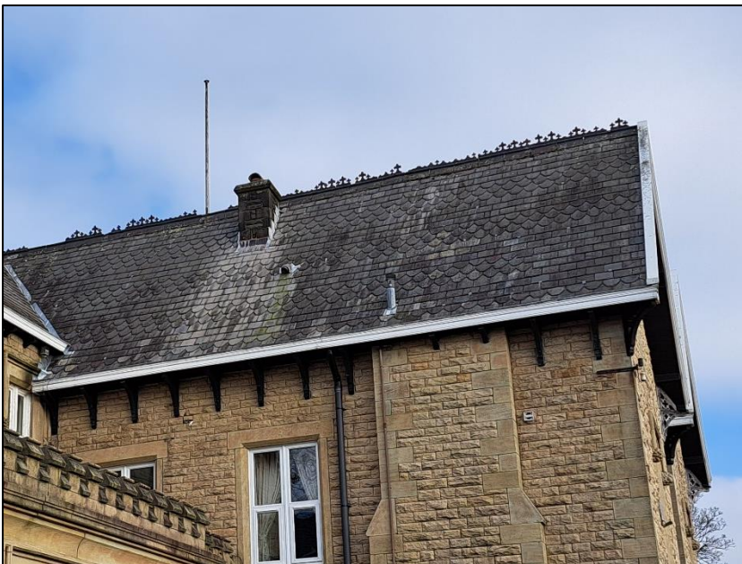
Photograph 4 showing a section of the roof
