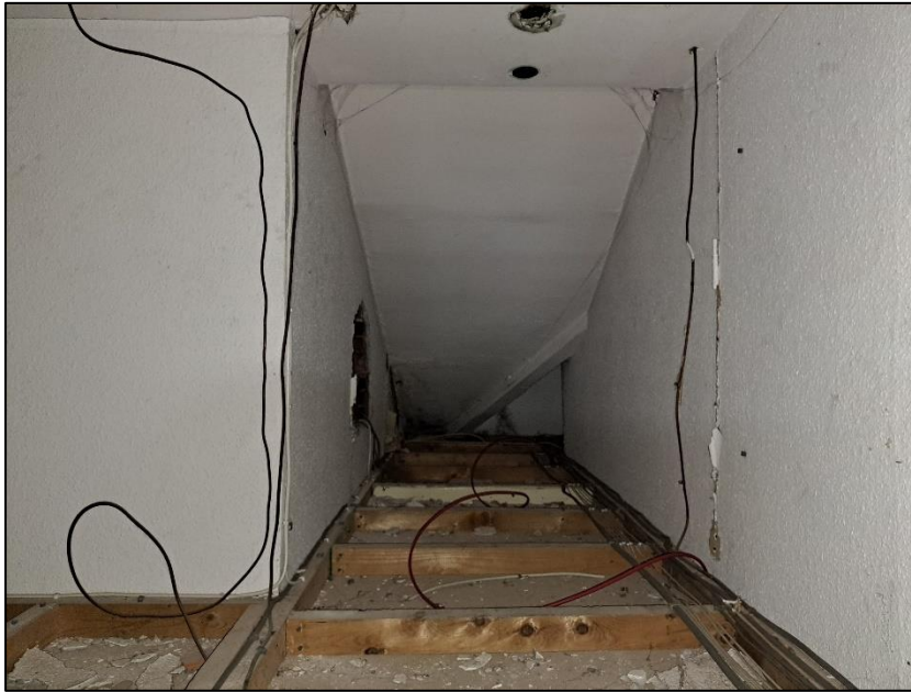
Photograph 13 showing the space above the false ceiling
