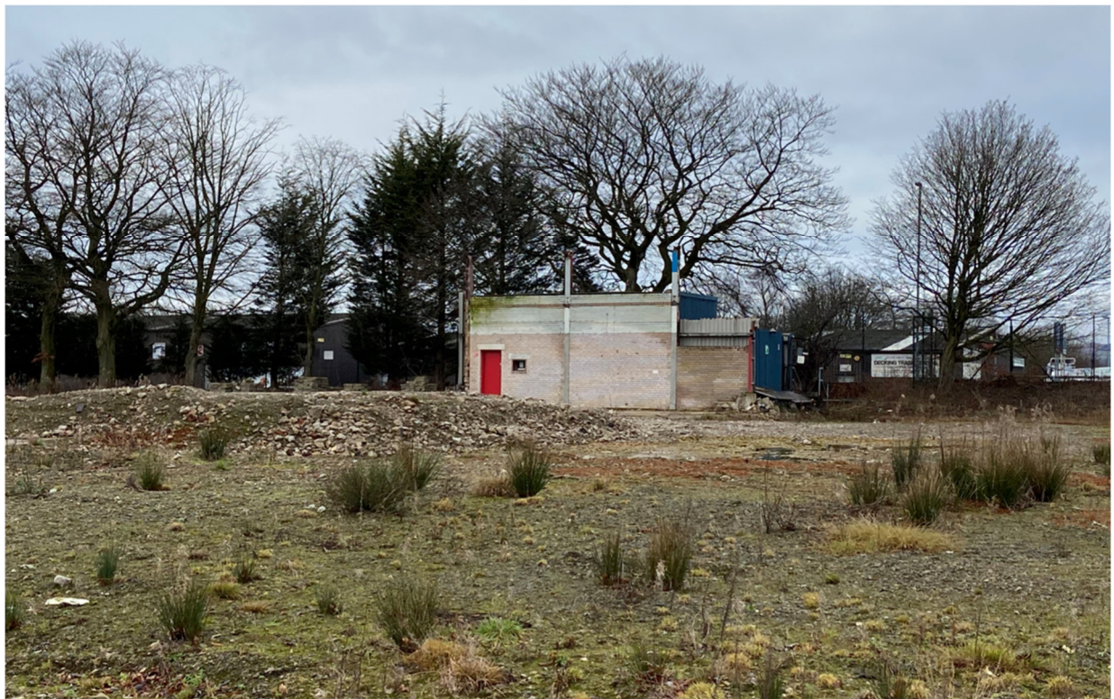
Photograph 5 – General site photo looking north.
