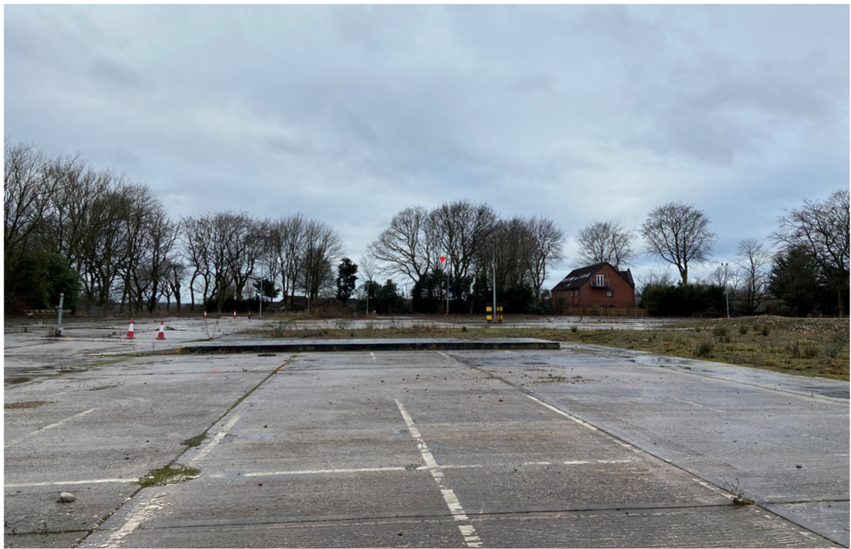
Photograph 1 – General site photo looking North West.
