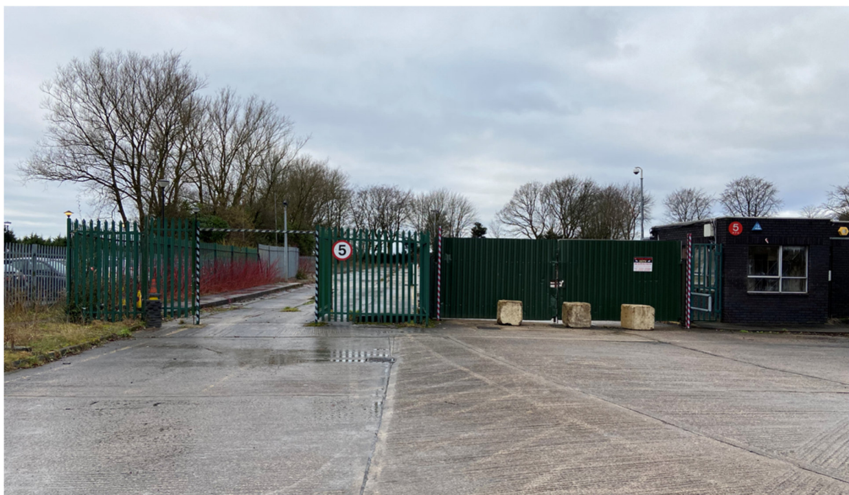
Photograph 6 – General site photo of access gate.
