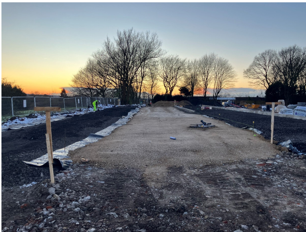
Photograph 4 – Forming of Roads
