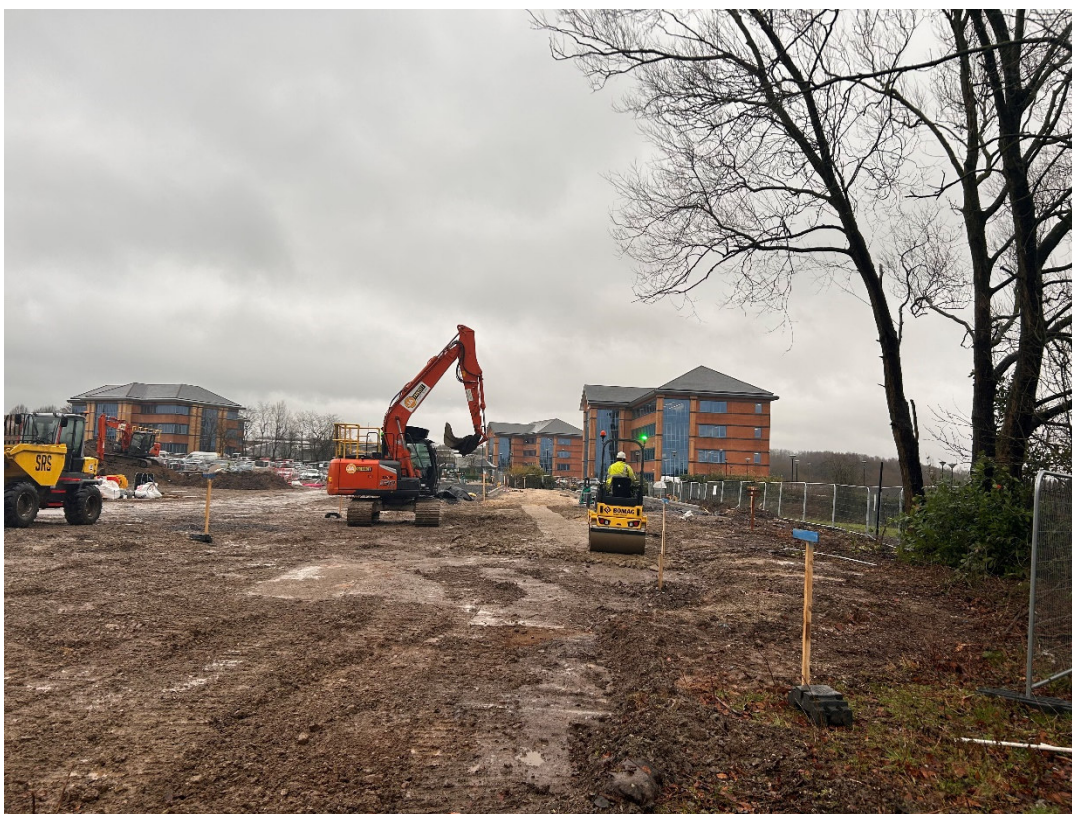
Photograph 3 – Compaction of Formation Level
