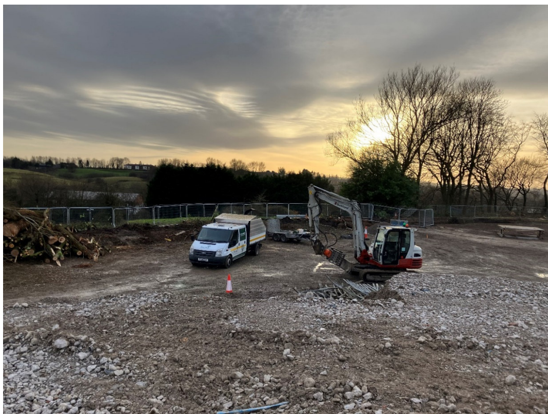
Photograph 1 – Area of devegetation following removal of trees
