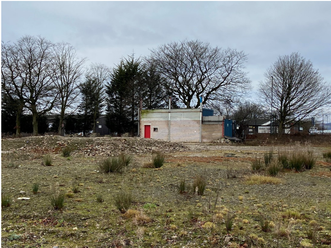
Photograph 5 – Existing building on site.
