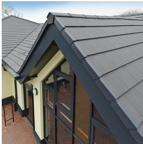
Roof. Dark grey concrete slates
