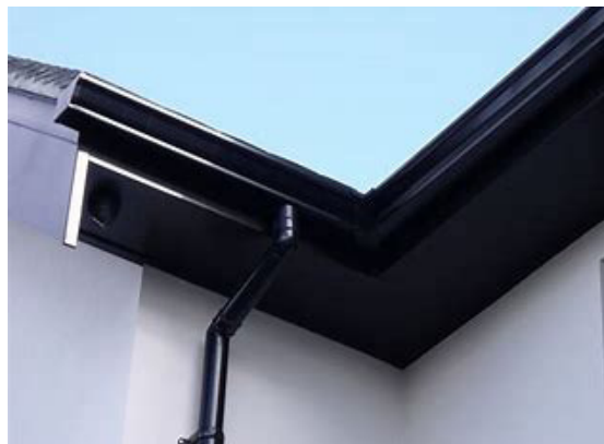
Black UPVC fascias & rainwater goods
