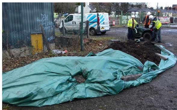
Sheeting of contaminated materials
