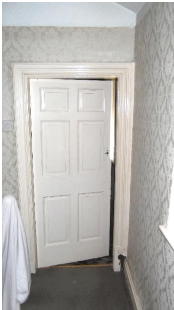
Original 6 panel door and frame. Wall removed in hall.
