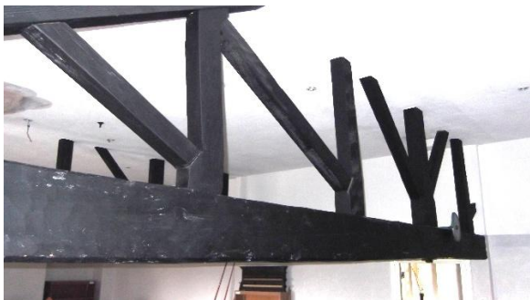
Truss at second floor.
