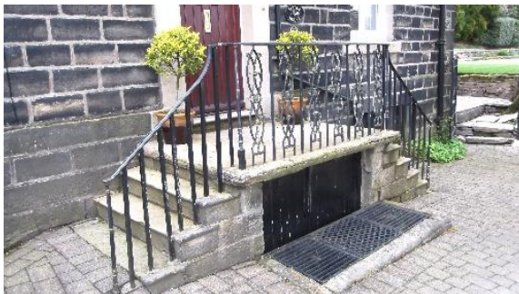
Steps, balustrade and boarded doors beneath.
