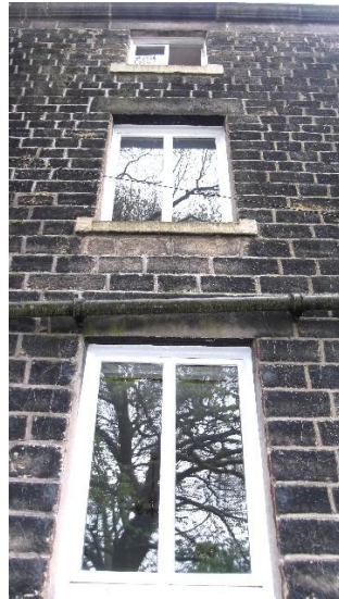
Main entrance and casement windows
