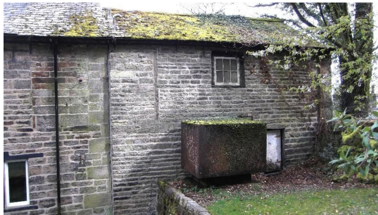
Rear of barn showing possible blocked-in doorway (behind the downspout) to main house and stones positioned vertically.
