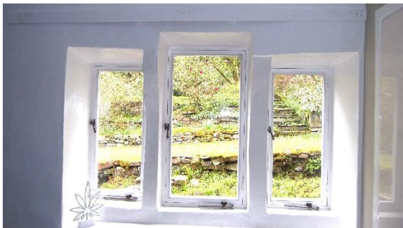
First floor rear window.
