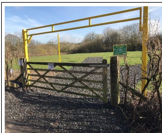
Photograph 1: Site access from Woodhill Road with height restriction
