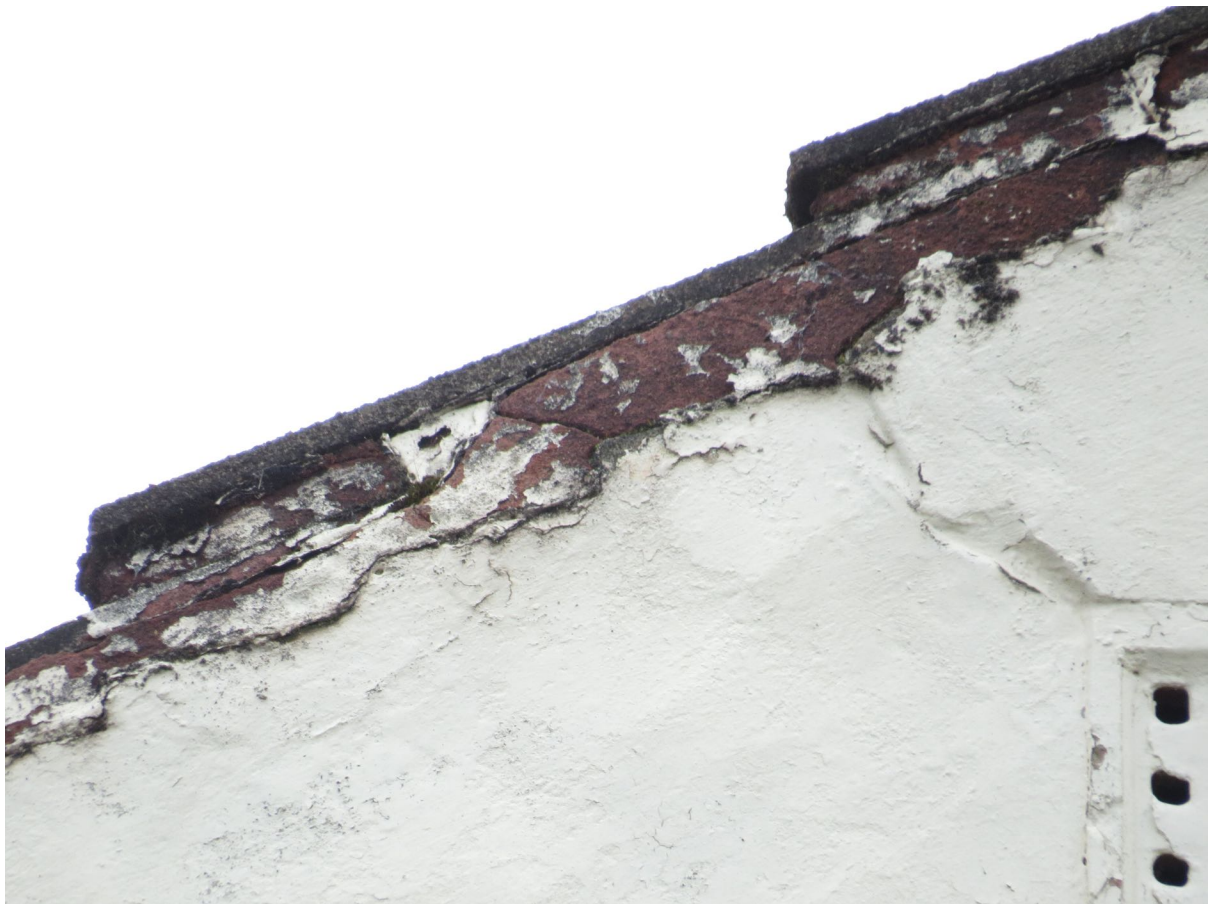
8 – Cement at the verges is intact with no suitable gaps.
