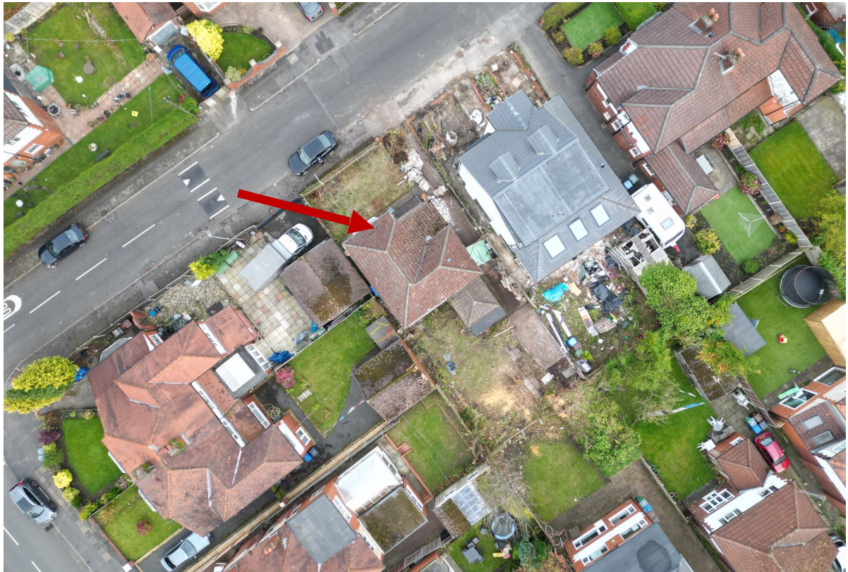
1.6b – 2 Windsor Road – aerial photograph.
