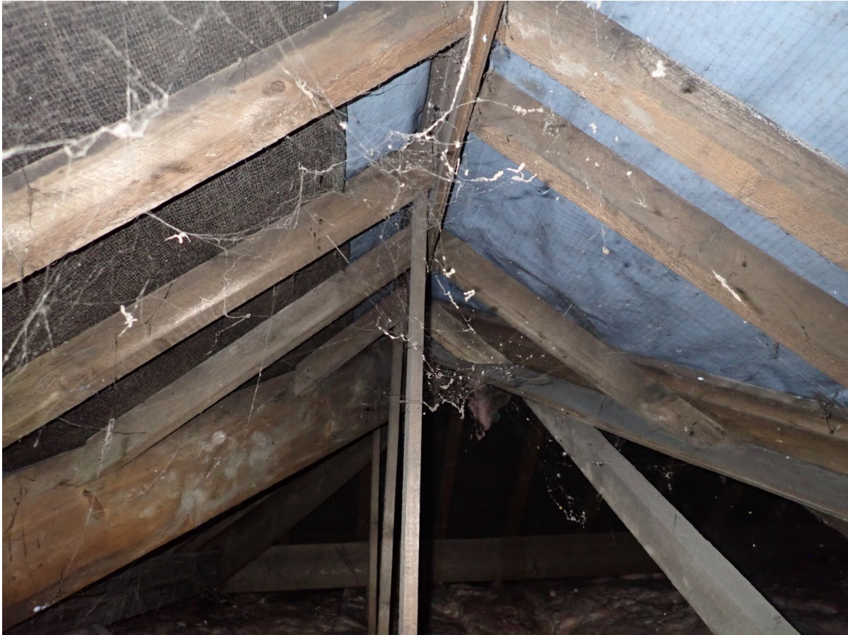
3.2a – The roof void.
