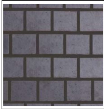
02. Brickwork Detailing Forterra 'blue smooth' brick laid in header bond with light grey mortar, bucket handle finish
