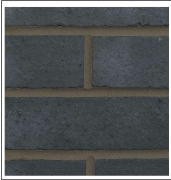
01. Brickwork Forterra 'blue smooth' brick laid in stretcher bond with light grey coloured mortar, bucket handle finish
