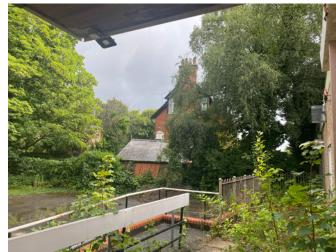
The western elevation of No.27, viewed from the entrance of the library.
