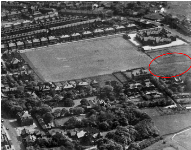
Aerial photograph showing Pinfold Lane. The site location is highlighted in red.
