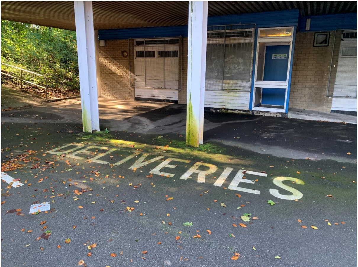
Figure 3.1 – Deliveries Area (Looking South) (Source: Curtins site visit, 9 th September 2025)
