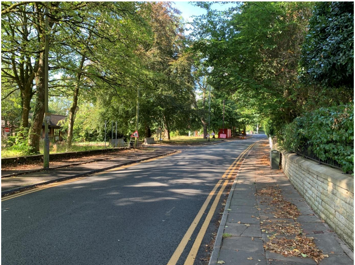
Figure 3.5 – Pinfold Lane, East of Site Access (Looking West)
