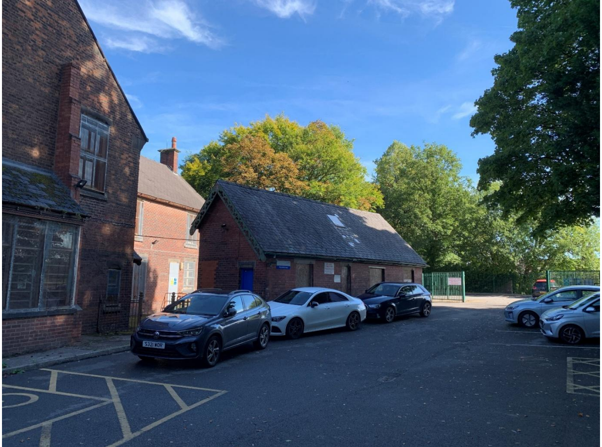
Figure 4.7 – Parking Adjacent Main Entrance (Looking Northeast)
