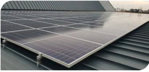
Figure 4. typical rooftop PV
