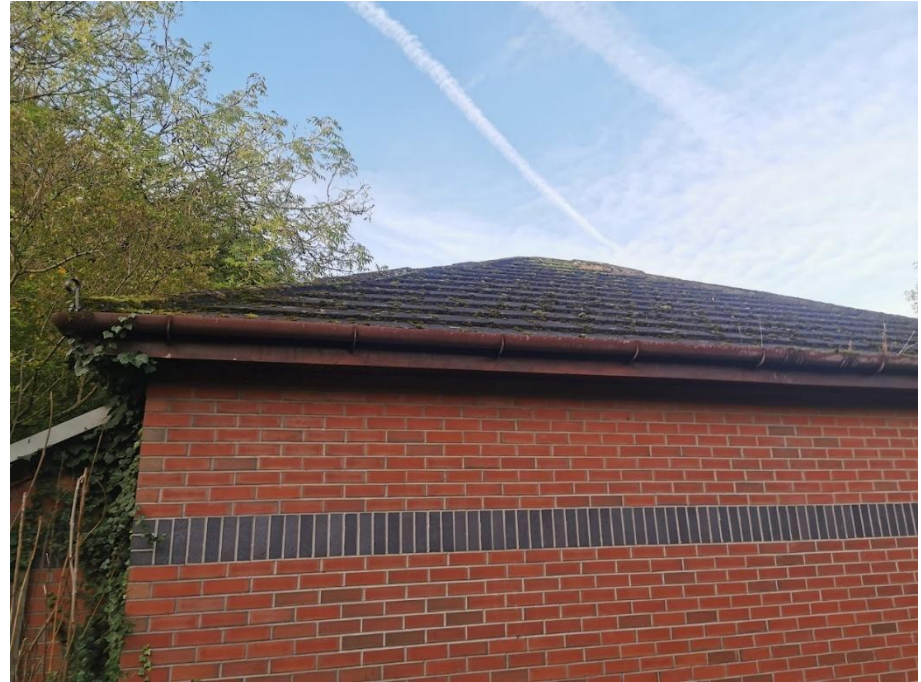
Photograph 14- Well sealed tiles on B2
