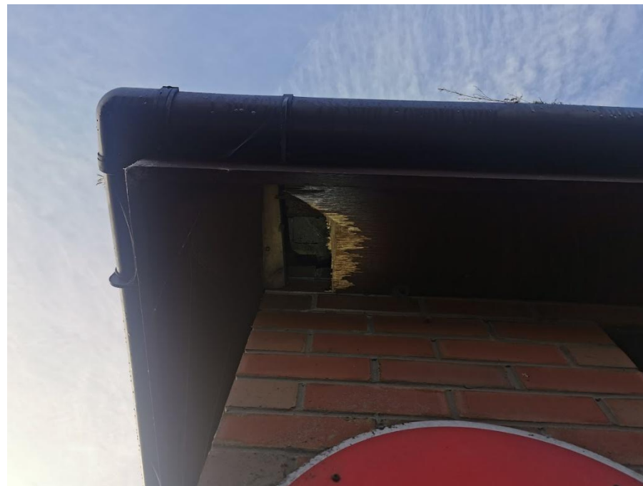
Photograph 12- Soffit feature on B2
