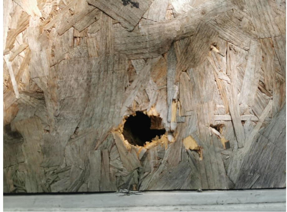
Photograph 6- Potential window gap on southern elevation
