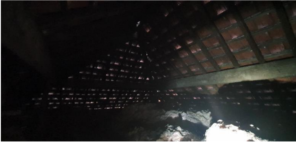
B1 – loft area looking south east (pictured above).
