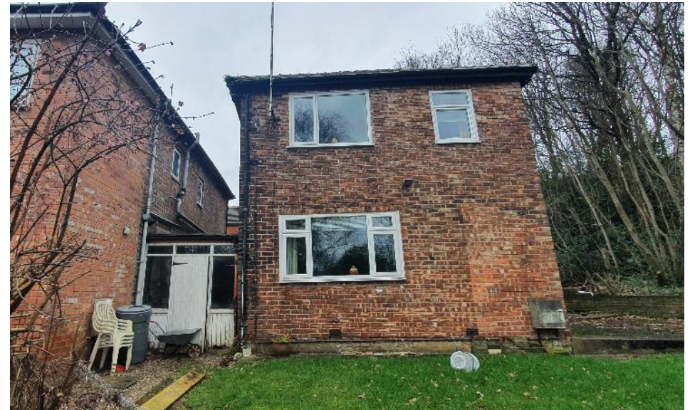
B1 – south eastern elevation (pictured above).
