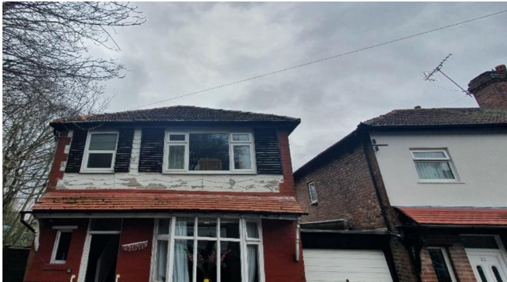
B1 – north western elevation (pictured above).
