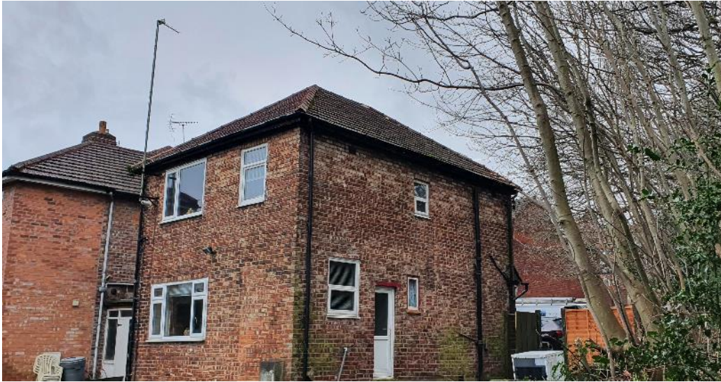
B1 – northern and eastern elevations (pictured above).
