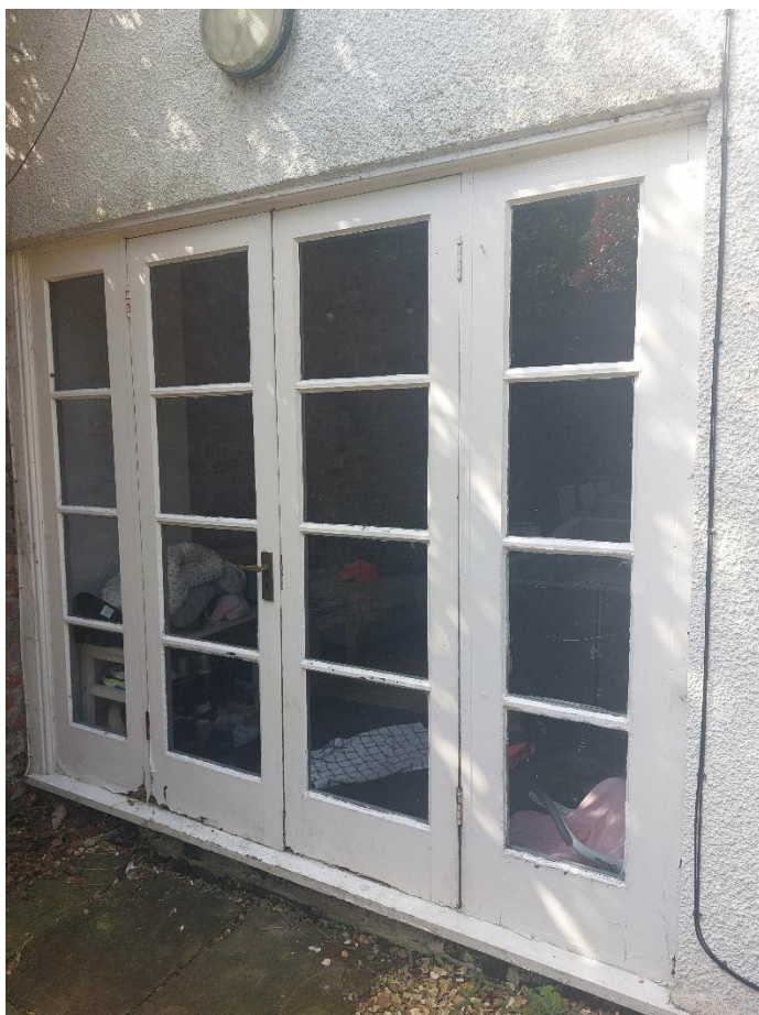
Figure 13: Lower Ground Floor Kitchen Door/Window
