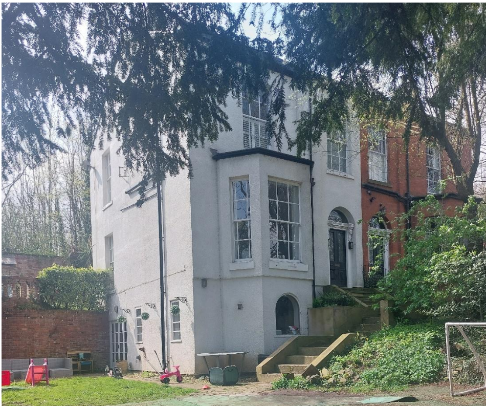
Figure 4: 17 Prestwich Park Road South front and side elevation – from within the garden.
