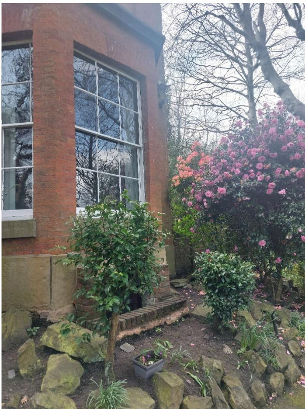
Figure 10: No.19 front bay window – lower ground floor mostly beneath ground
