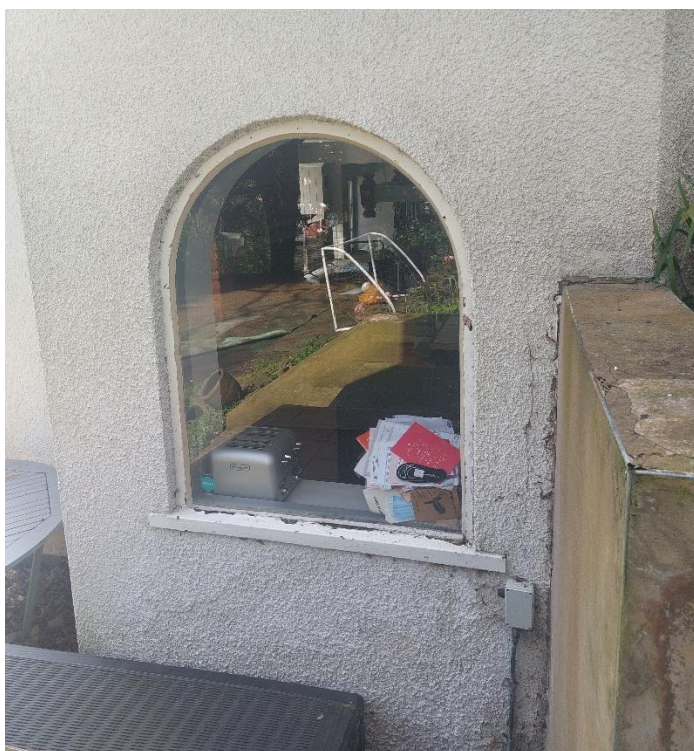
Figure 7: Lower ground floor front window
