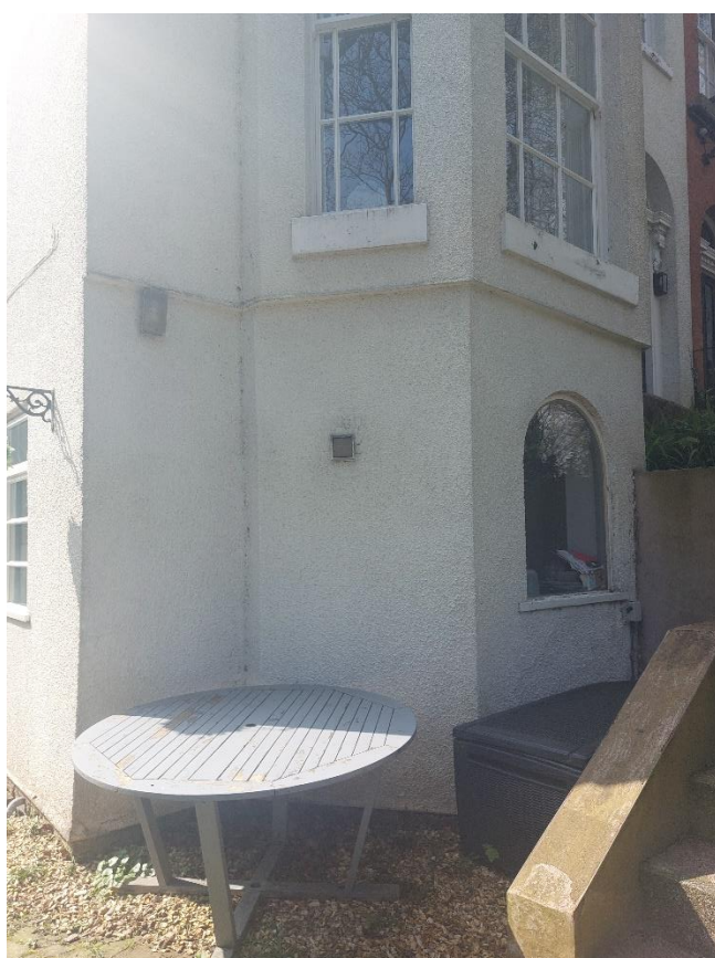
Figure 8: Lower ground floor front window and bay
