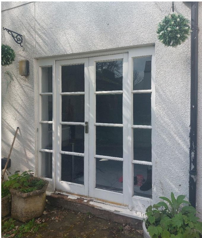
Figure 16: Upper Ground Floor Kitchen Window/Door
