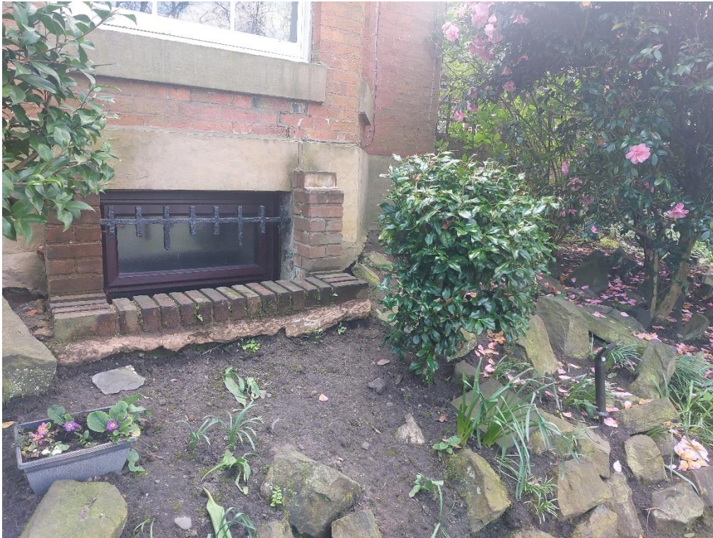
Figure 11: No.19 front bay window – lower ground floor mostly beneath ground
