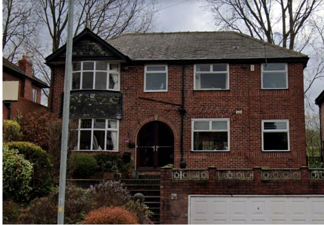
Extended dwelling at no. 49 Hilton Lane
