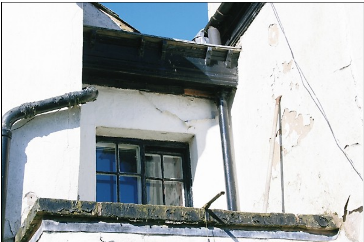
14. Sliding 12-pane stairlight above porch
