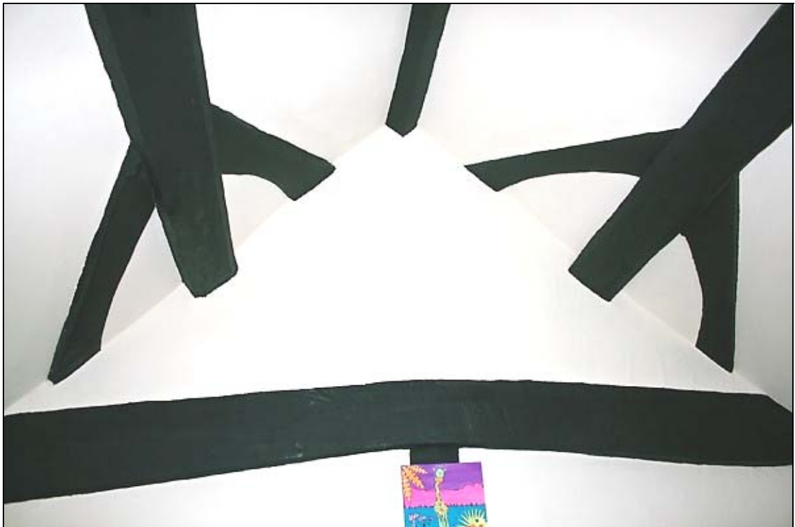
40. Purlins and windbraces of concealed truss at junction of centre wing bedroom and hall
