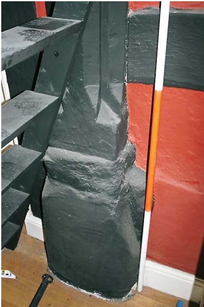
25. West wallplate north of truss 2 showing pegs for close studding
