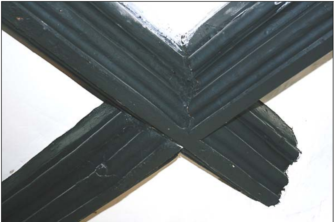
36. Moulded beams in ground floor bathroom, probably late 15 th -early 16 th century. Because they die into the crosswall, it shows the room they belonged to extended to where the kitchen is now
