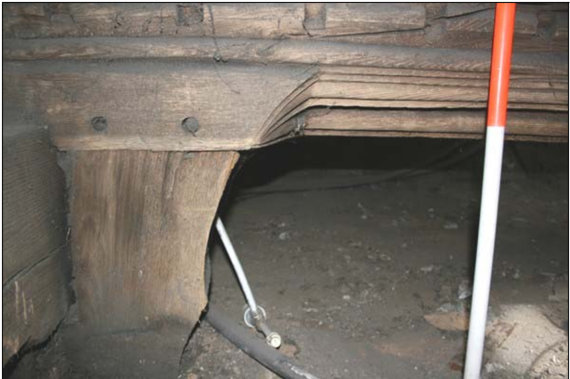
29. Detail of moulding on dais truss tiebeam and scalloping of west wallpost head
