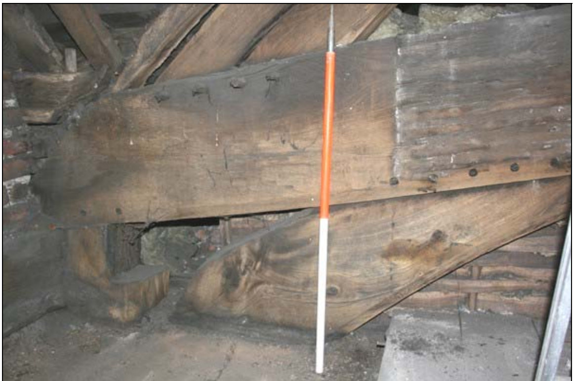
24. Detail of arch-bracing at east end of truss 2 tiebeam
