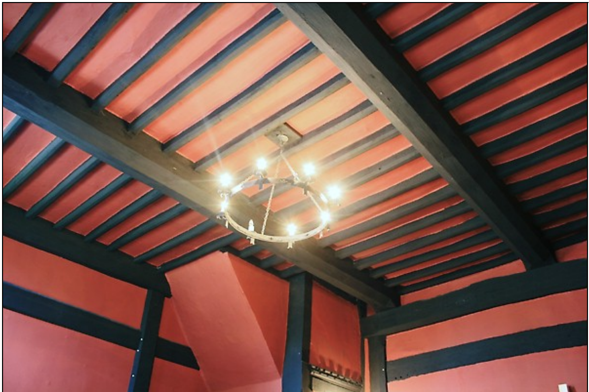
19. Inserted ceiling of hall on deep chamfered beams carried by secondary framing
