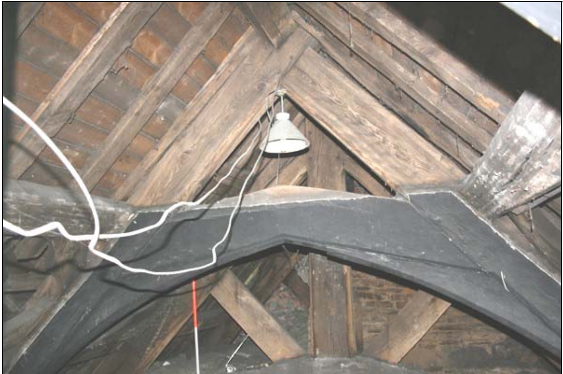
27. Truss 3, an arch-braced collar truss. Blackened area is where it was formerly exposed and stained (see Plate 20)
