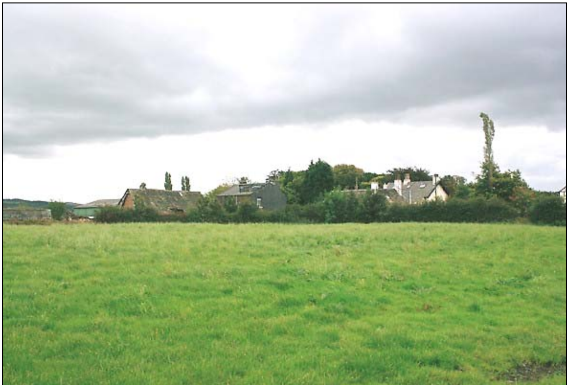
1. Setting: the Brandlesholme group from the northwest, showing, left to right, cruck barn, Brandlesholme Farm, Brandlesholme Old Hall and Brandlesholme Hall
