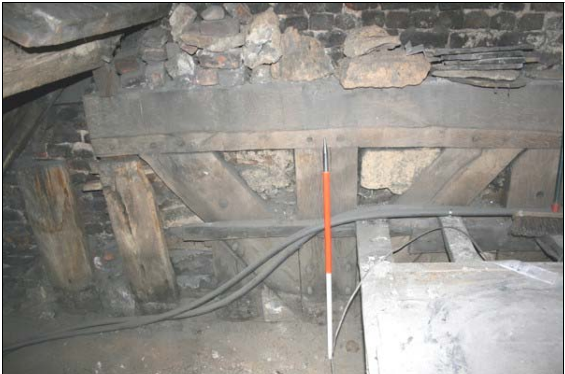
32. North end wall of hall showing termination of west end of tiebeam of former fifth truss; wallpost and truss replaced by handmade brick. This probably occurred when solar wing was truncated, leaving this wall exposed
