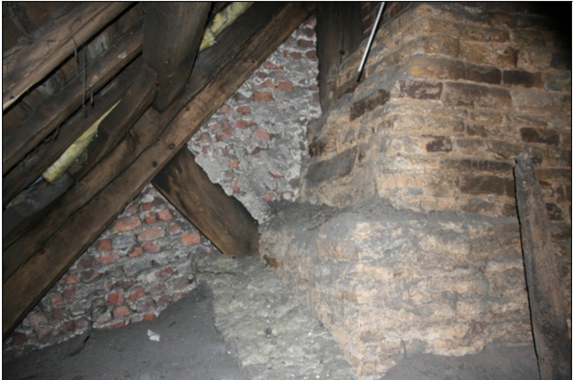
21. Exposed portion of spere truss, now buried in crosswall with Brandlesholme Old Hall
