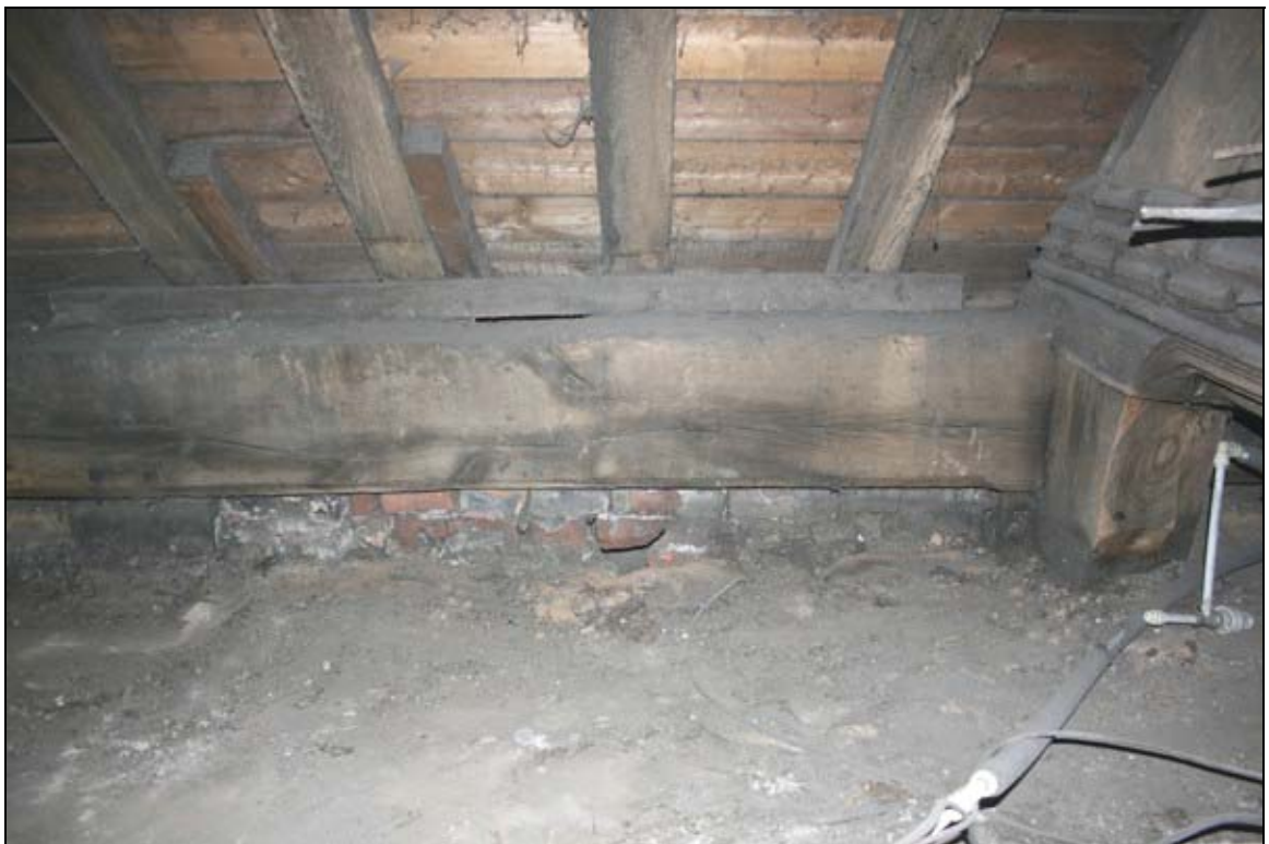
34. West wallplate south of truss 4, where lack of peg holes for close studding suggests presence of window
