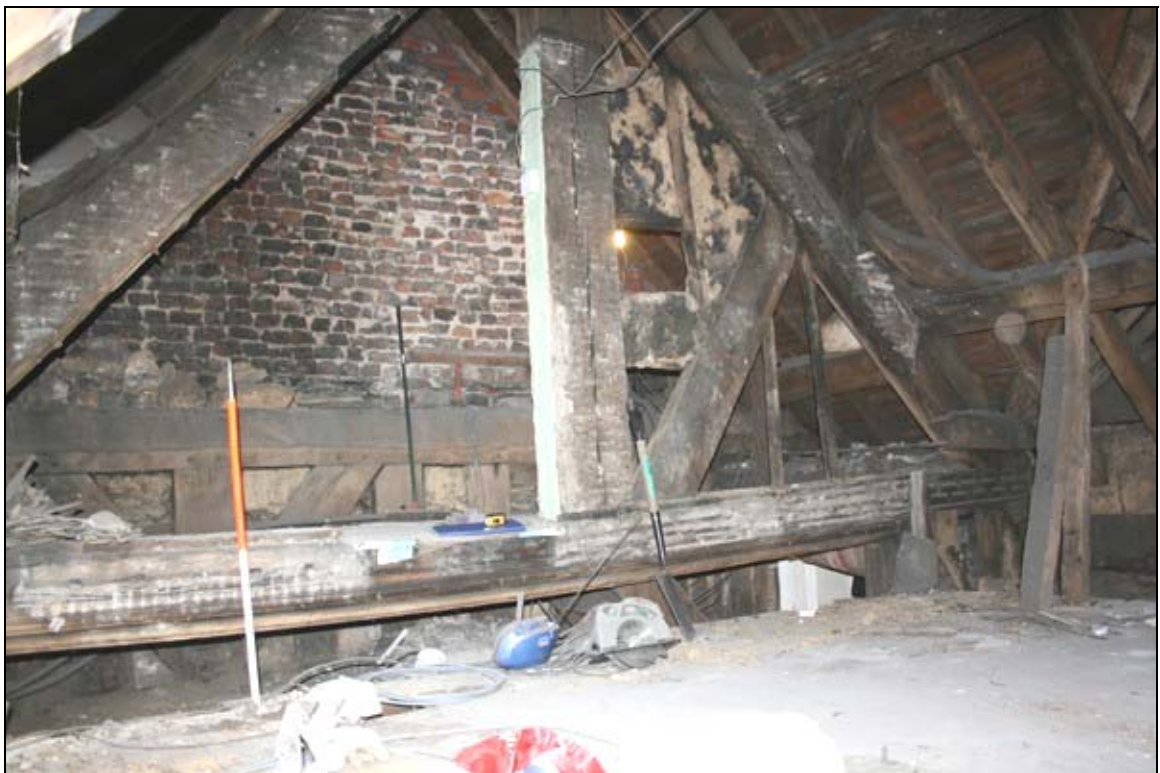
28. Truss 4, originally over dais, with west brace later removed to facilitate access to attic
