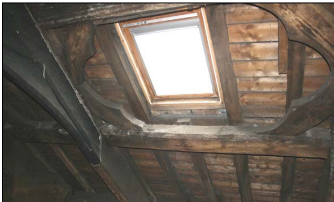
41. Existing rooflight in attic, showing relationship with common rafters and boarded roof
