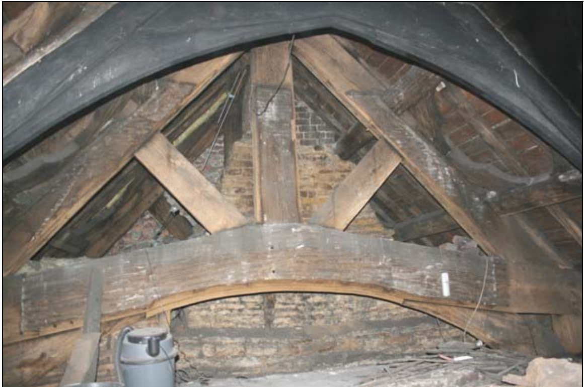
11. General view of trusses above former open hall. Centre of image is kingpost truss in front of inserted stack, with spere truss partly visible where embedded in crosswall beyond; in foreground is part of arched-braced truss
