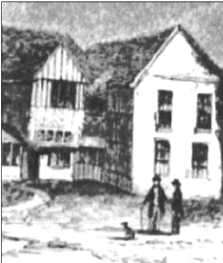
10. Enlargement of 1844 illustration showing close studded return wall of crosswing and on centre wing, latter also with herringbone framing
