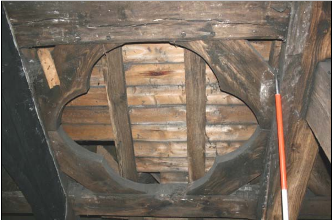
33. Detail of quatrefoil windbracing, between trusses 2 and 3 on east side
