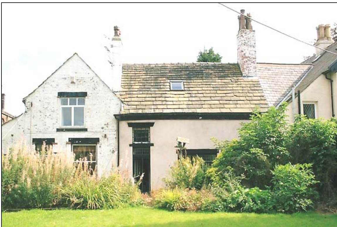
9. Rear (west elevation) showing kitchen and outshut on left, and main range followed by Brandlesholme Hall on right. Below: map evidence showing how kitchen and outshut were added between 1891 and 1908; probably during alterations of the latter year.
