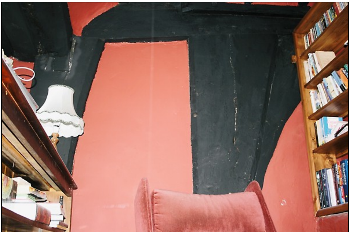
22. Wallpost (left) and spere post with arch-bracing exposed in minstrel's gallery
