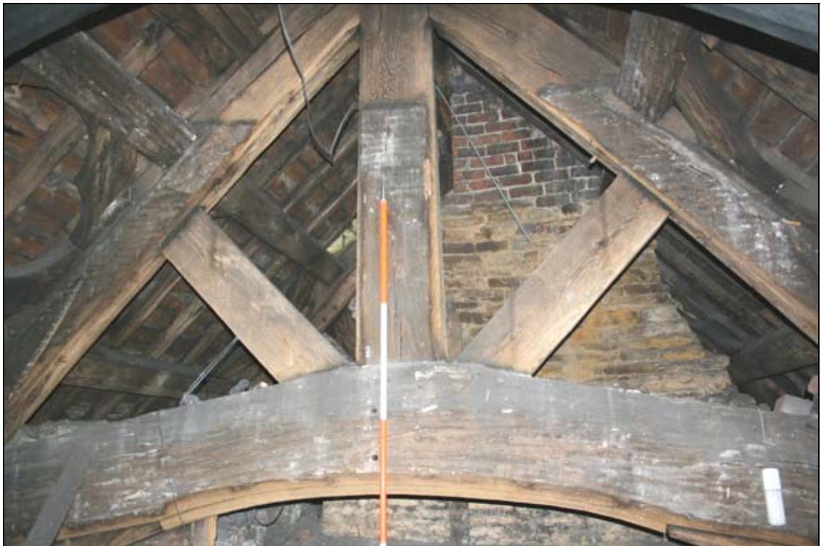
23. Truss 2, with braced kingpost and cambered arched braced tie
