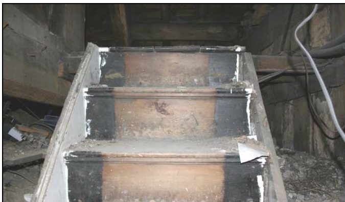
42. Staircase in attic, showing relationship to dais truss (left) and close-studded north wall (right)
