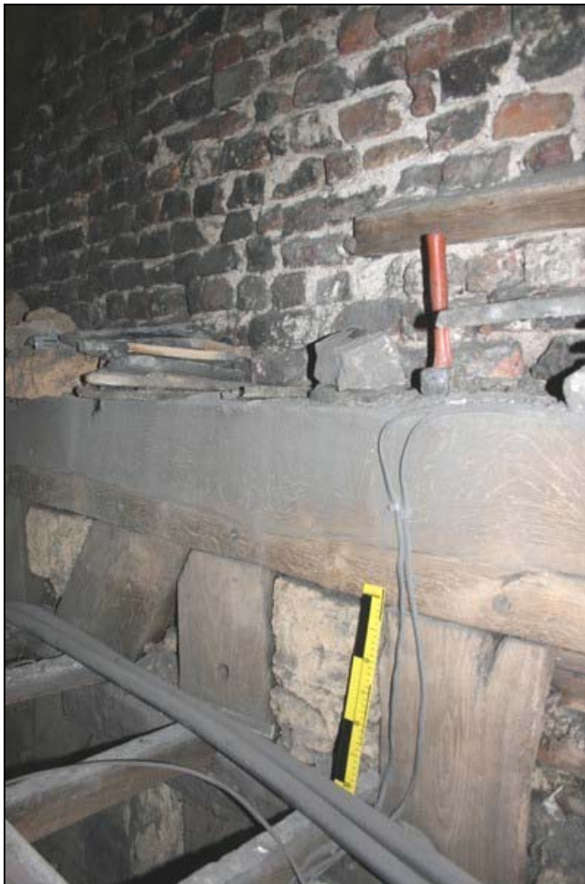
11. General view of trusses above former open hall. Centre of image is kingpost truss in front of inserted stack, with spere truss partly visible where embedded in crosswall beyond; in foreground is part of arched-braced truss
