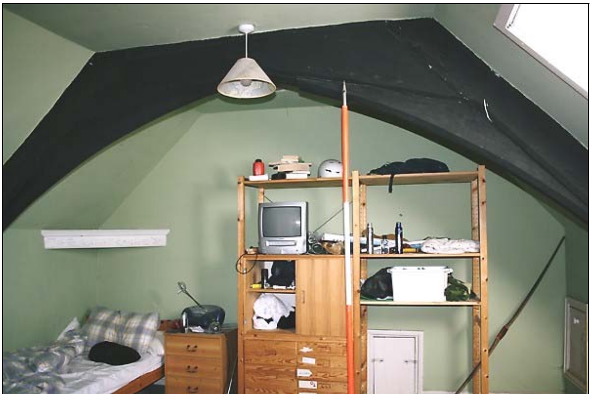
20. View of attic before removal of lath-and-plaster partitions of circa 1908, showing arch-braced truss (For present view see Plate 27)
