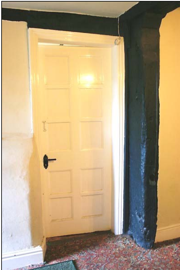
35. Ten-panel late 17 th or early 18 th century door to centre wing. Battered lobby wall, probably originally external and of stone, to its left
