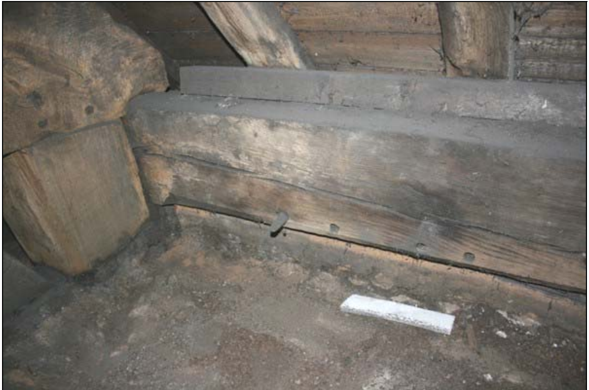
25. West wallplate north of truss 2 showing pegs for close studding
