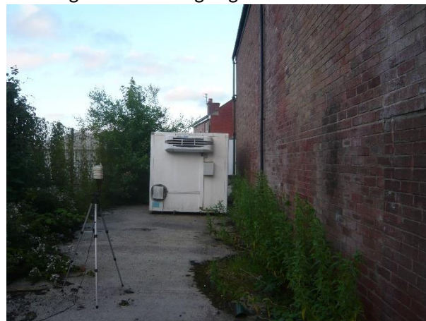
Photo 4: Northern elevation of the building, cabin, hard standing, colonising vegetation and scrub
