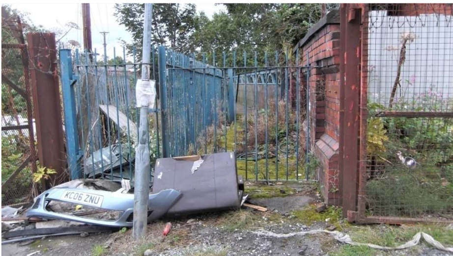
Former bridge access ramp, Milltown Street
