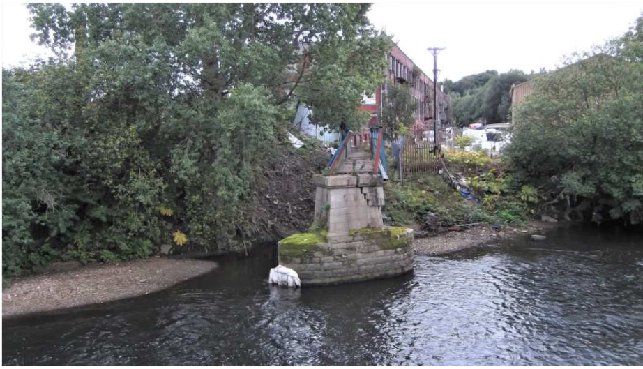
Central pier viewed from Rectory Lane.
