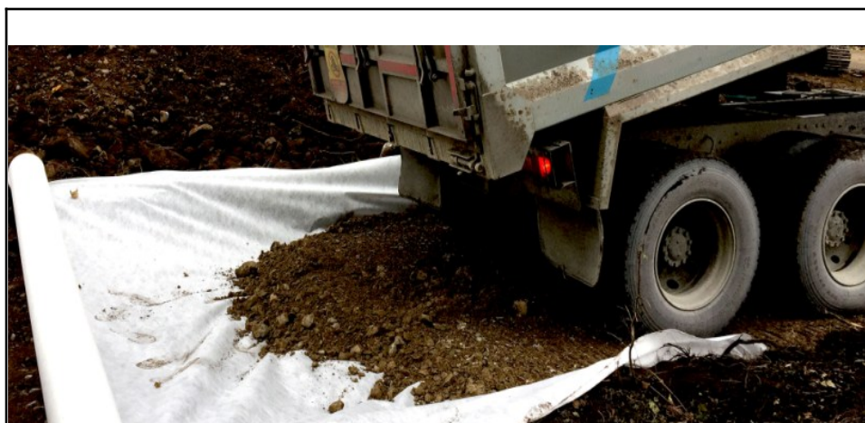
Terram over the clay which will prevent weed growth.
