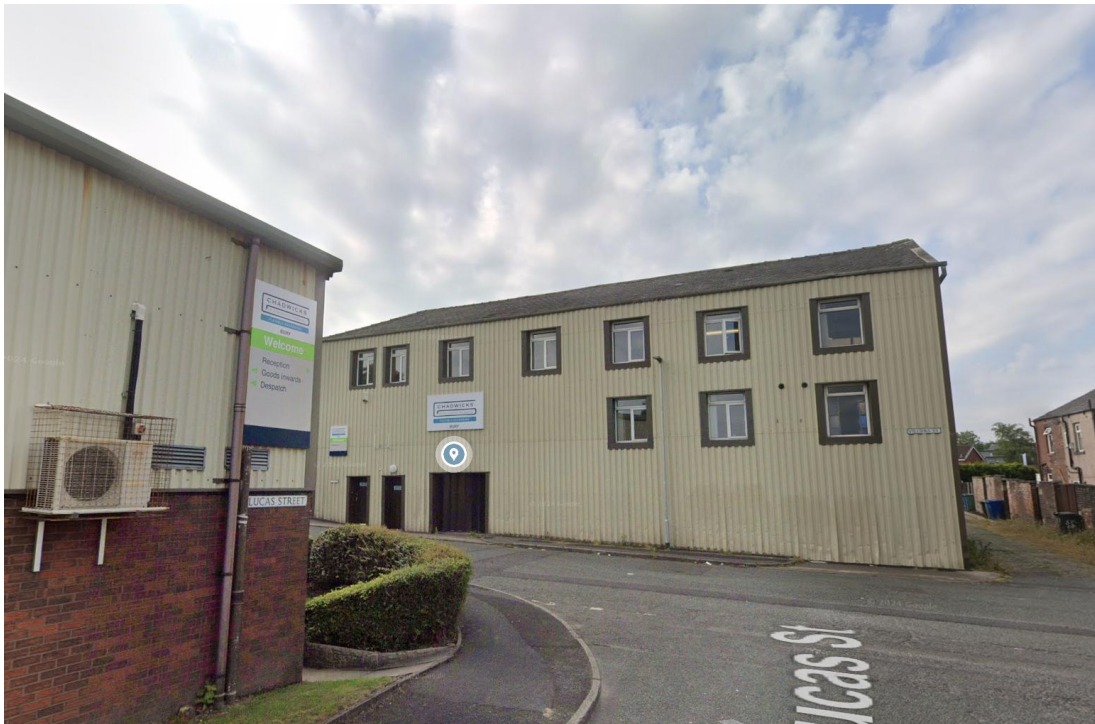
D01 Chadwicks Administration Building, Existing Window Precedent
