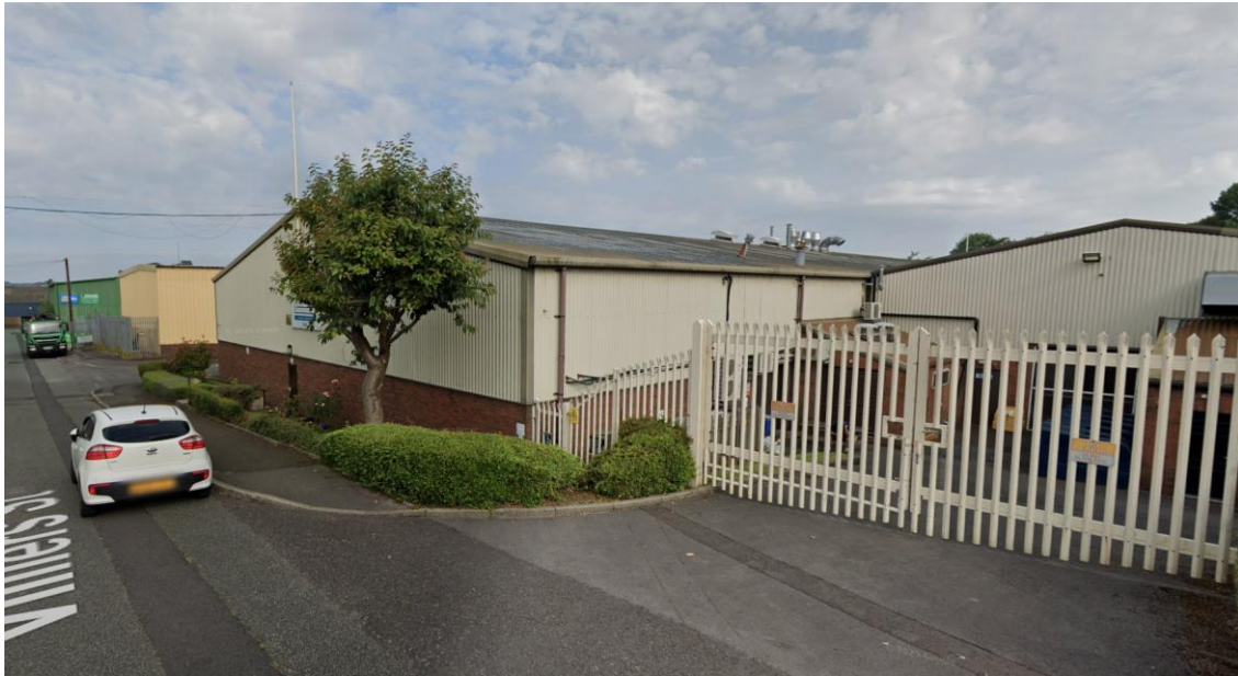
B04 Existing east elevation and car park / loading bay
