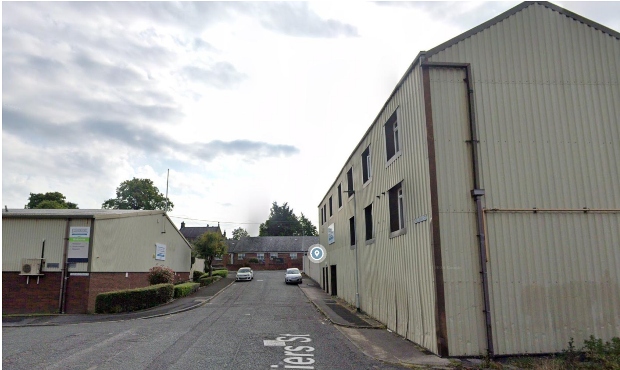
B06 View towards Chadwicks administration building to the south
