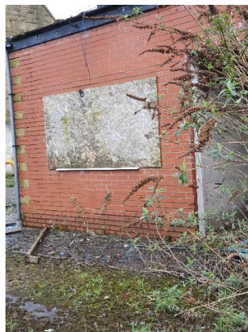
B2 Ground floor boarded up window in 2020
