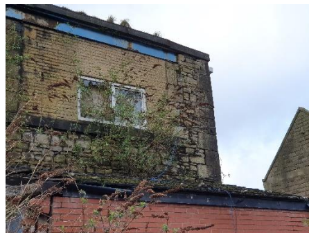
B2 Supporting beam to the eastern elevation in 2020
