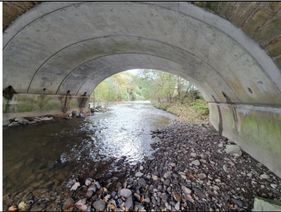
Photograph 7: Under the bridge north of survey Patch 5 of the River Irwell, October 2019.
