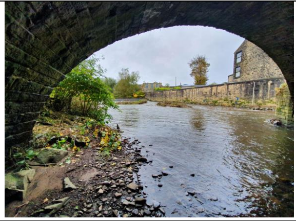
Photograph 8: Weir north of survey Patch 5 of the River Irwell, October 2019.
