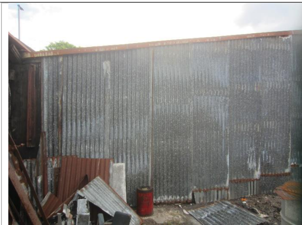
Photo 13: Eastern elevation of the lean-to
