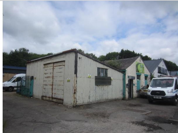
Photo 1: Lean-to and workshop bordered by hard-standing (taken from Bury Road)
