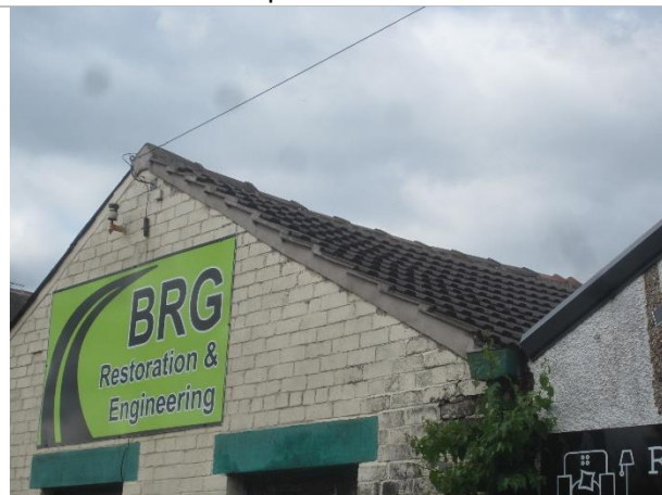
Photo 5: Eastern elevation of the workshop showing sealed roof verge and concrete tiles on north-facing pitch
