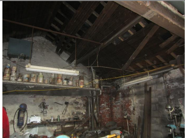
Photo 8: Interior of workshop
