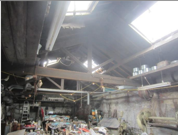
Photo 7: Interior of workshop with skylights
