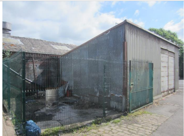
Photo 12: Eastern and southern elevations of the lean-to
