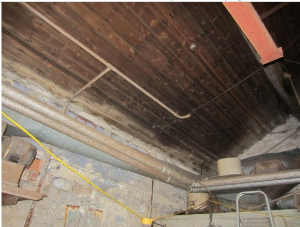
Photo 9: Interior of workshop with timber sarking
