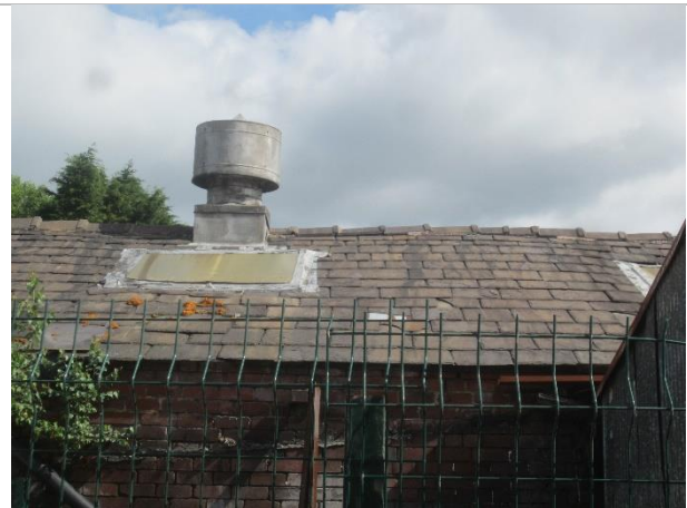
Photo 4: South-facing roof pitch of the workshop
