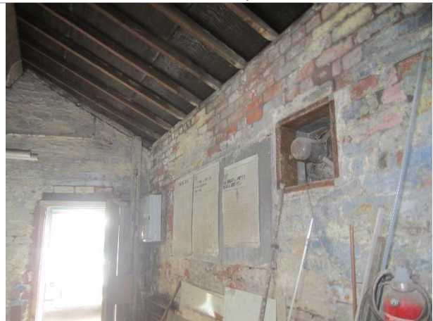
Photo 10: Interior of workshop
