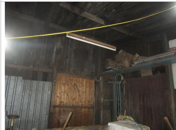
Photo 15: Interior of lean-to
