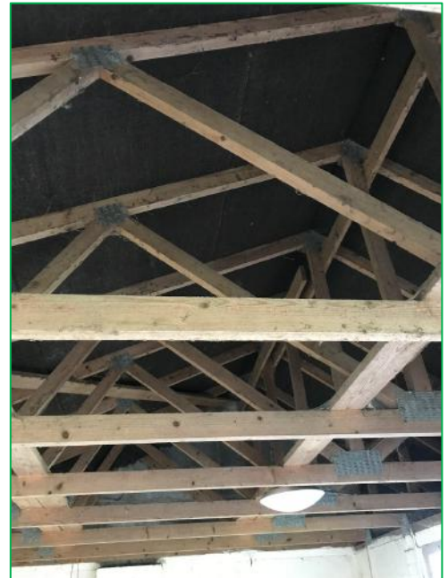
The internal roof structure with felt well-fitted
