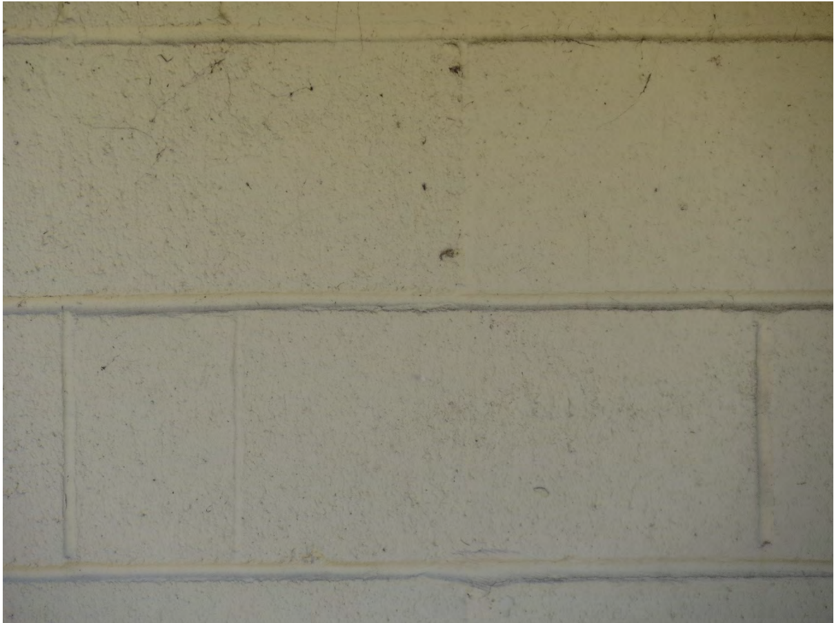
5 – Walls are in good condition with no gaps or cracks.
