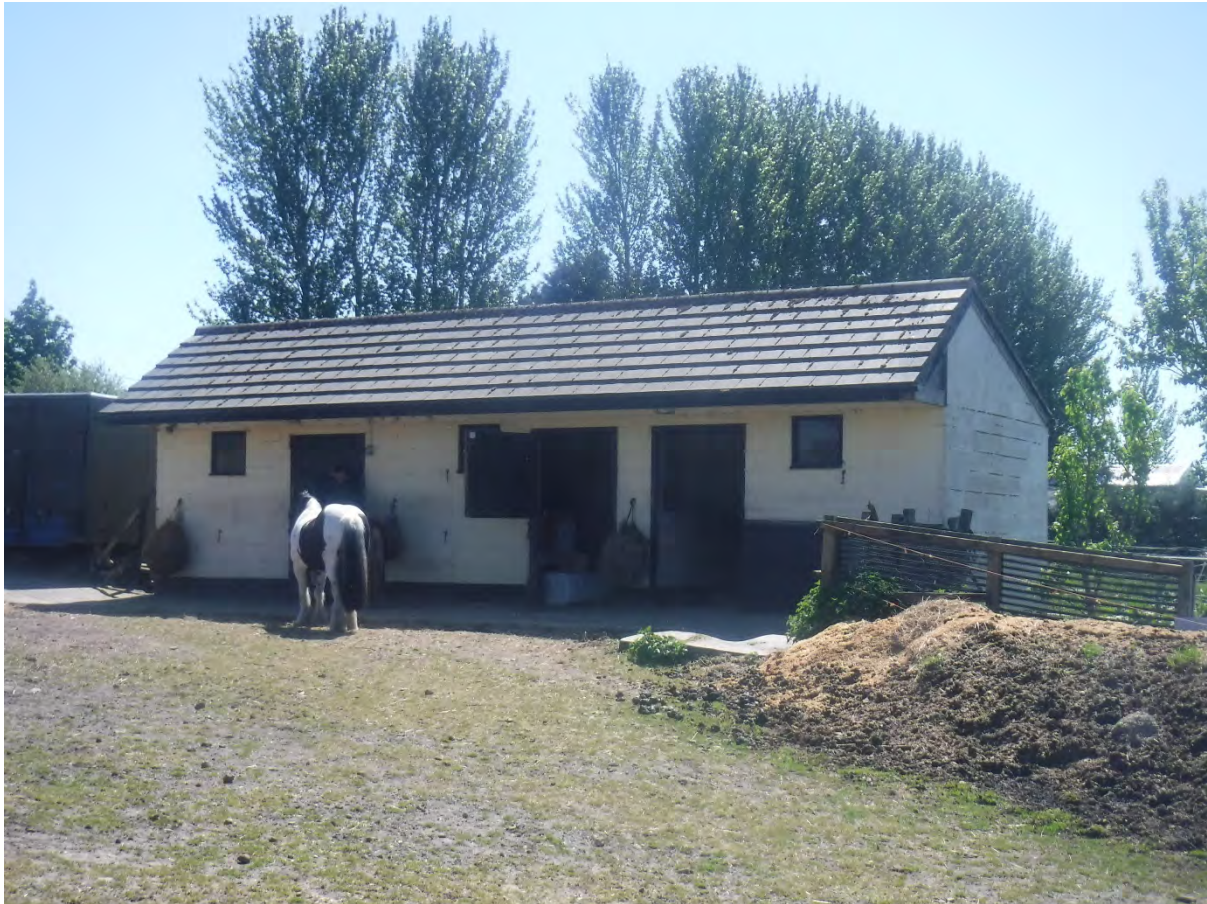
3.1a – The front of the stables.
