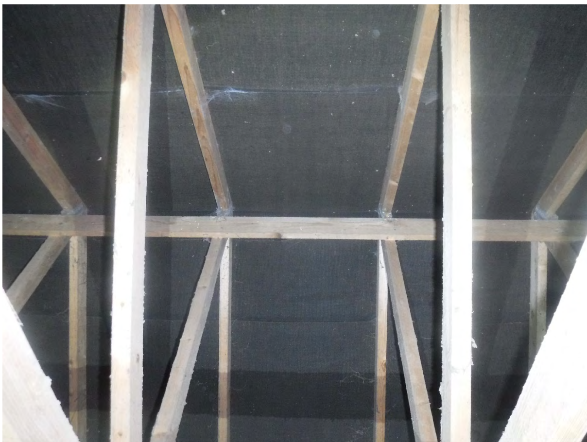
7 – The building has no enclosed roof void, and has a timber trussed roof structure.
