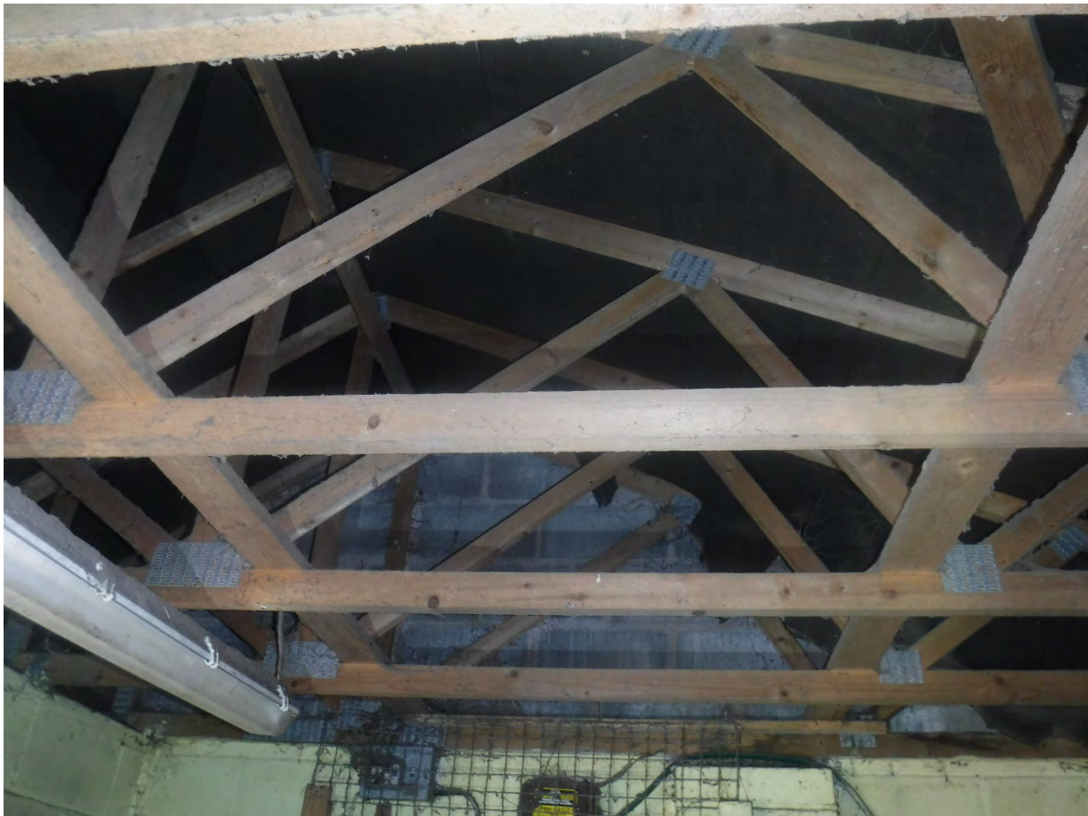
3.2a – The roof structure.
