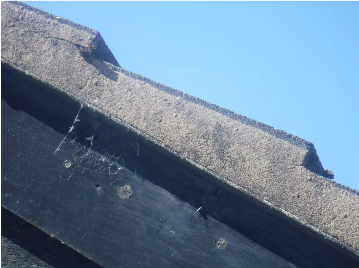
3 – Cement at the gable end verges is intact with no suitable gaps.
