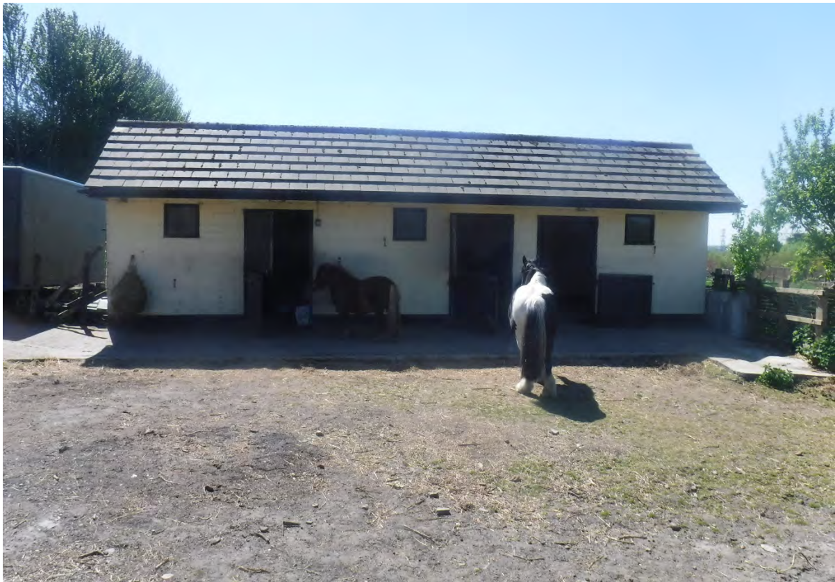
1 – The north facing front of the stable block.
