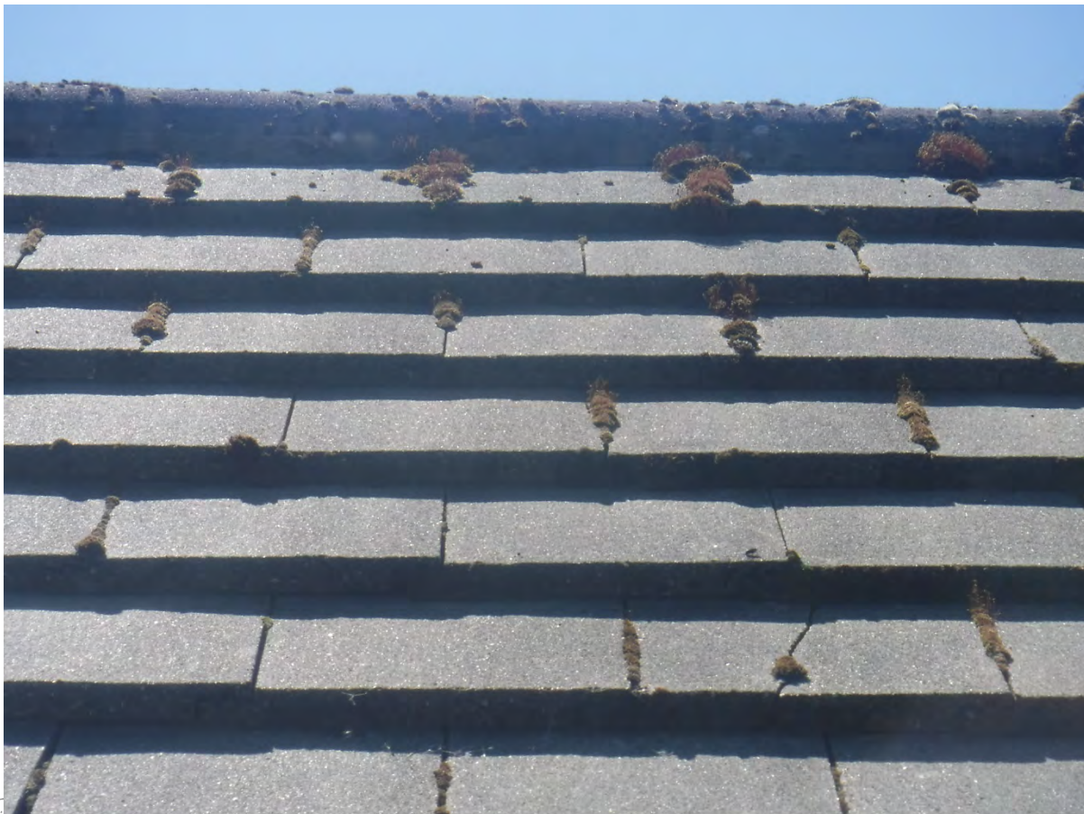
2 – Roof tiles are in good condition with no suitable gaps.
