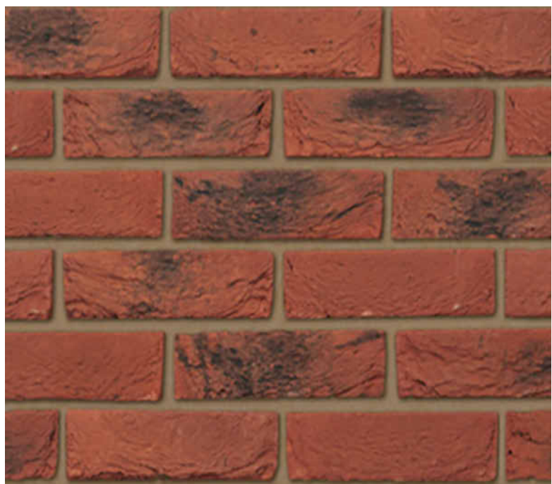
Brick Work - Rear Elevation
