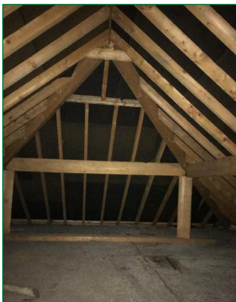
Showing the large loft void
