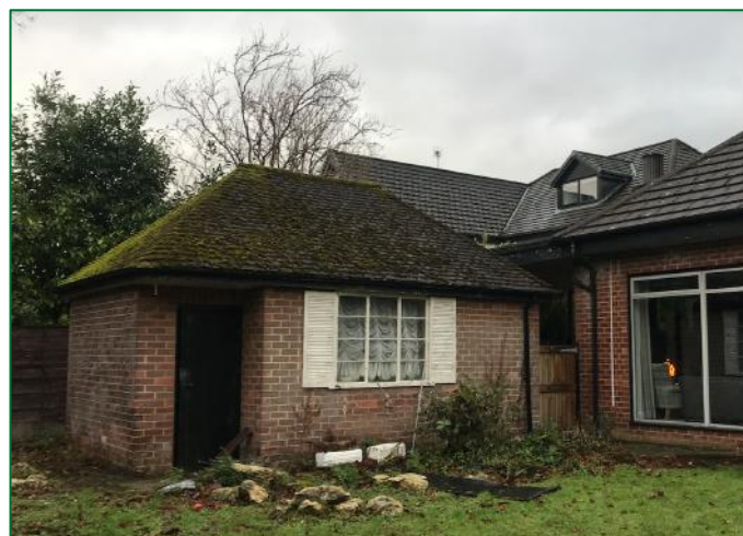
The northeast and southeast elevation of the garage
