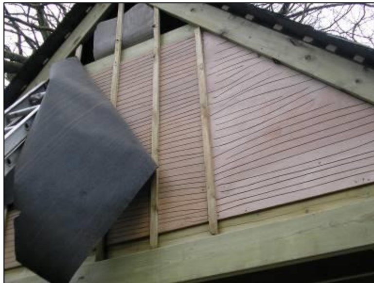
Arrangement of southern gable elevation coarse or grooved sheet timber, vertical battens and bitumen felt, horizontal battens followed by timber cladding
