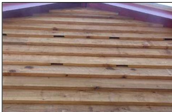
Figure 6.2 – Indicative cladding designs that will need to be installed on the southern gable elevation
