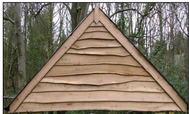
Figure 6.2 – Indicative cladding designs that will need to be installed on the southern gable elevation
