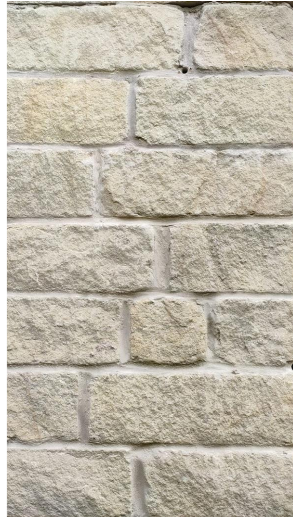
Rear Extension – Approved Planning Application 66471 Locally sourced natural stone
