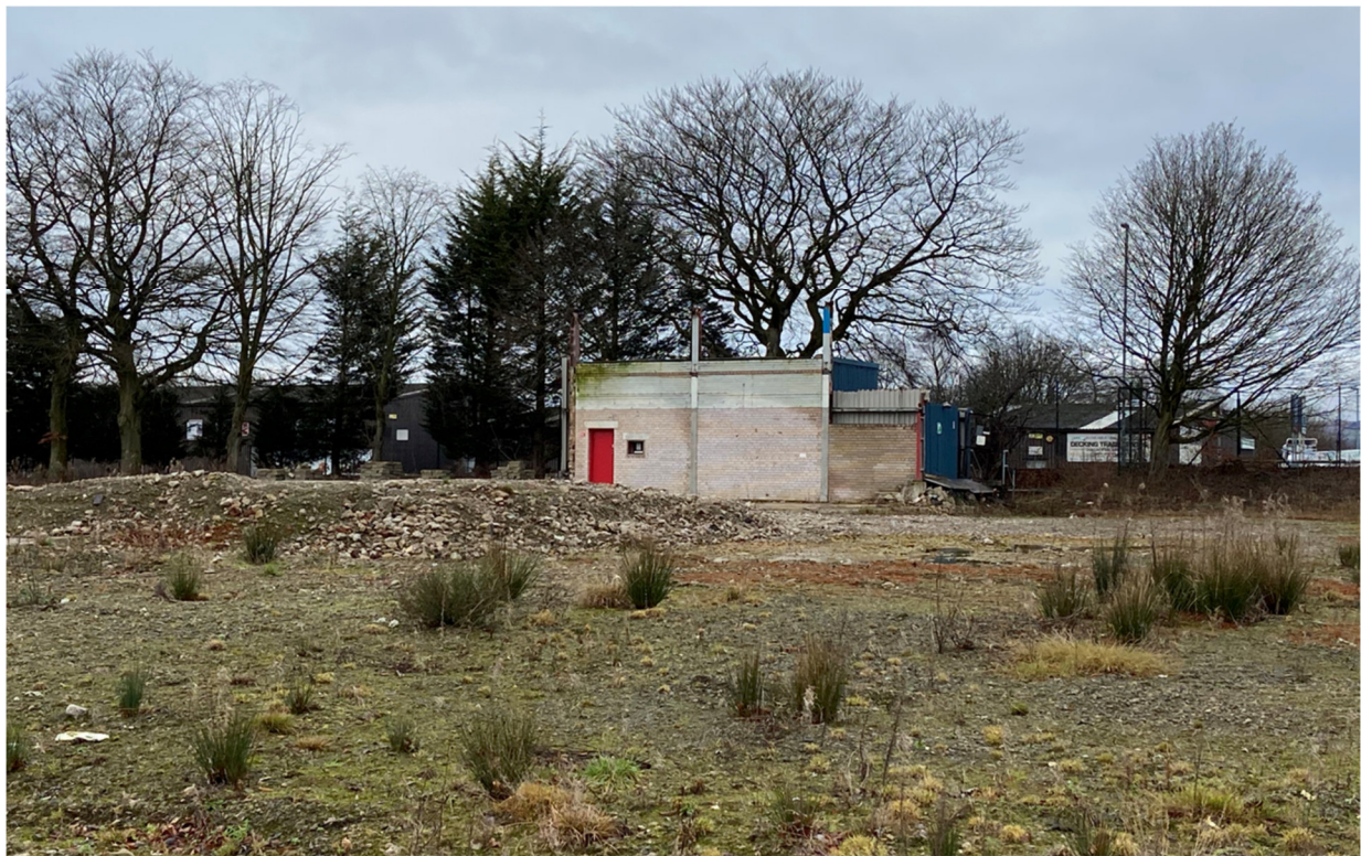
Photograph 5 – General site photo looking north.
