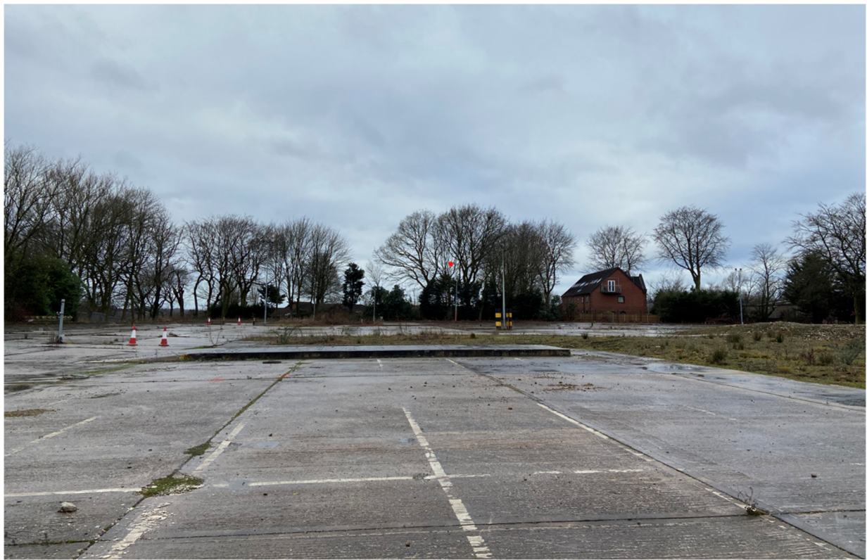
Photograph 1 – General site photo looking North West.
