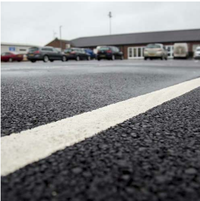
11. Permeable Asphalt - Parking 1 : 1
