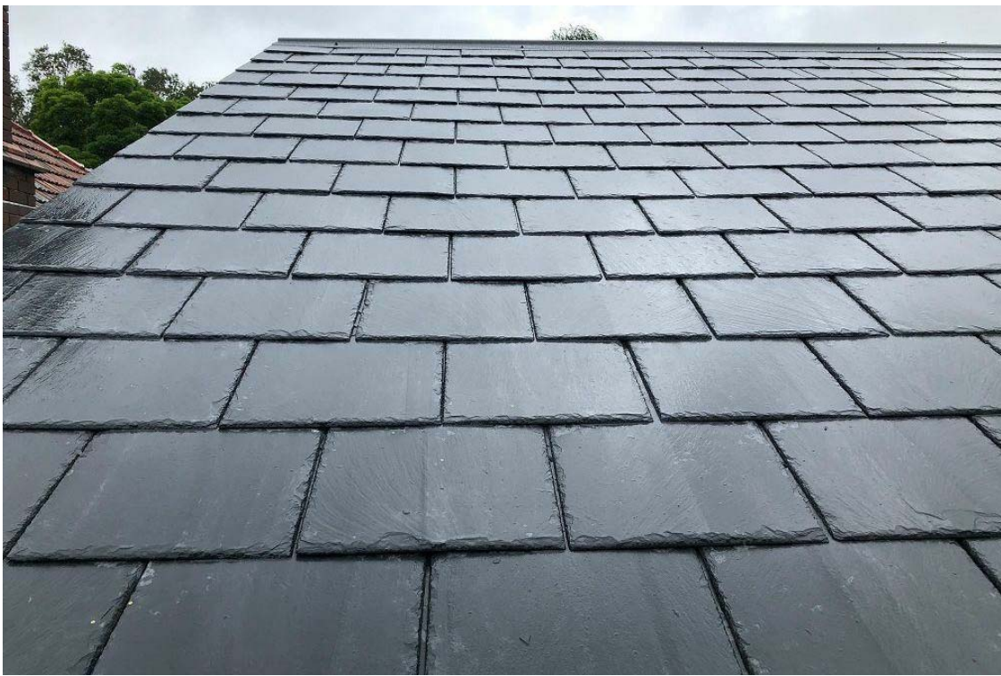
2. Natural Slate Roofing Tiles to Match Existing
