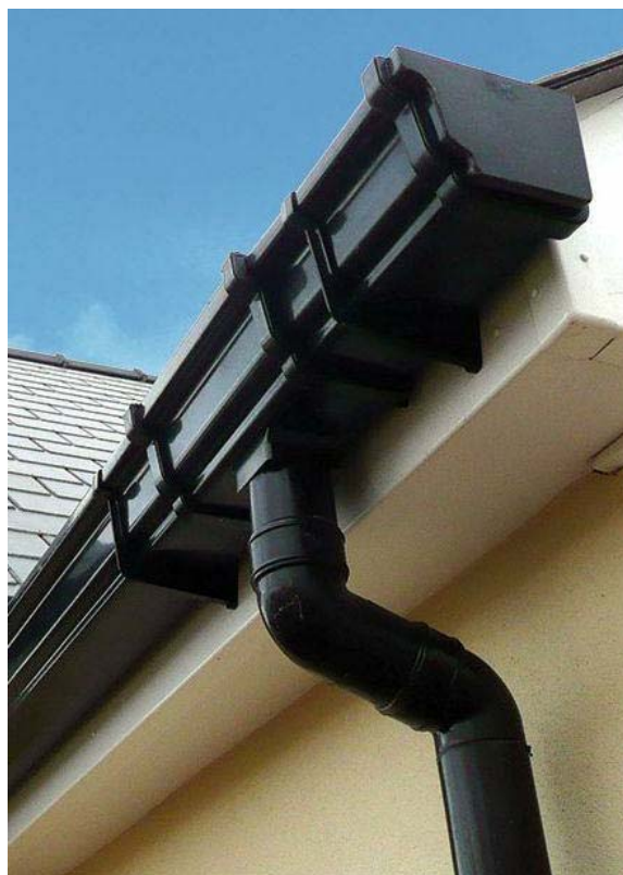
13. Black UPVC gutters and downpipes.
