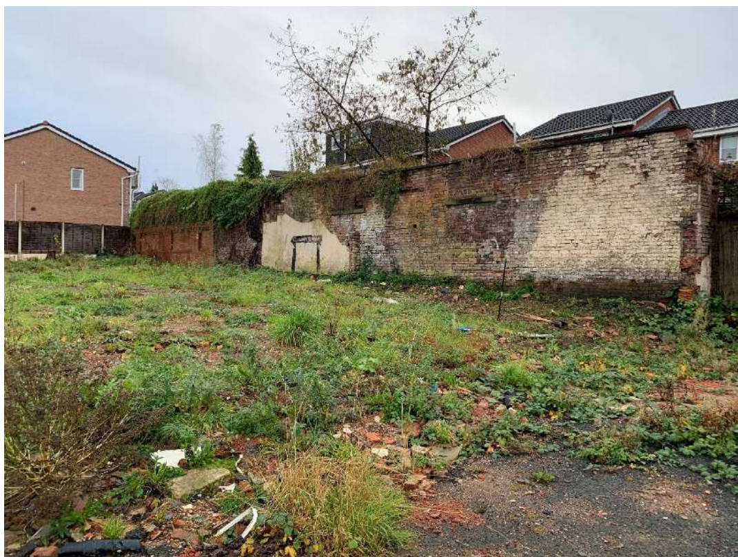
Photograph 16 – Retaining Wall On Southern Boundary
