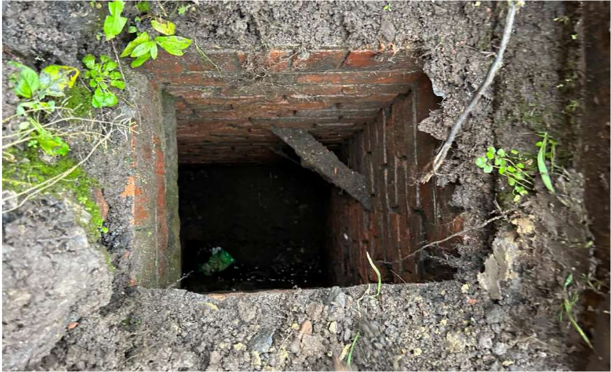
Photograph 19 – Manhole encountered in southern corner of site.
