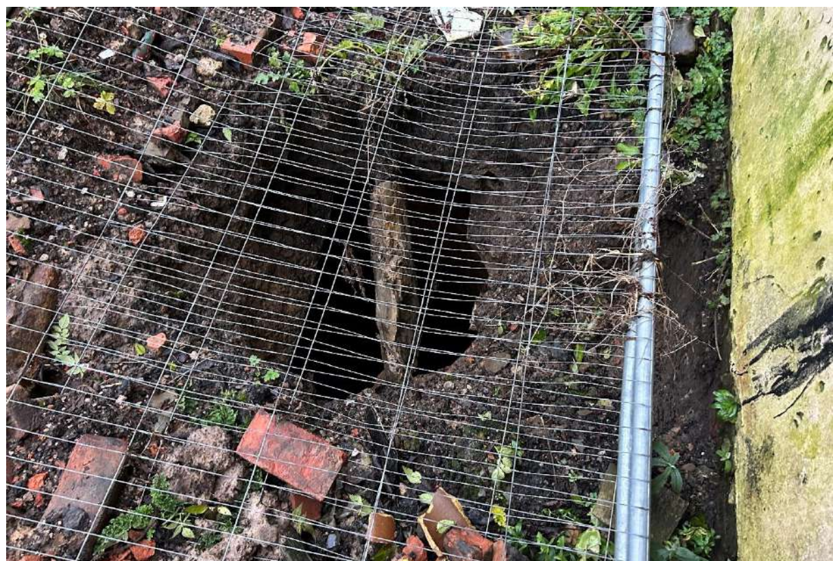
Photograph 26 – Current condition of well structure at surface.
