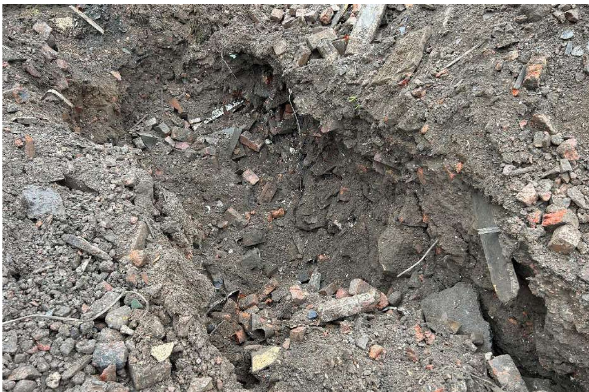
Photograph 23 – Instability of TP05.
