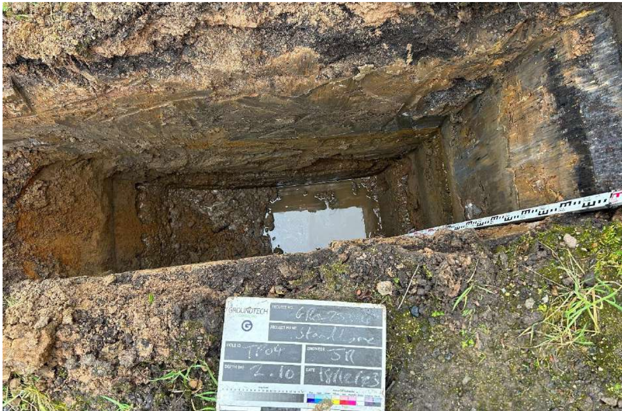
Photograph 21 – TP04 showing groundwater seepage at 1.60m bgl.
