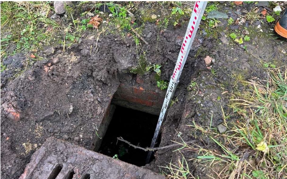
Photograph 20 – Manhole chamber depth is approximately 2.30m.
