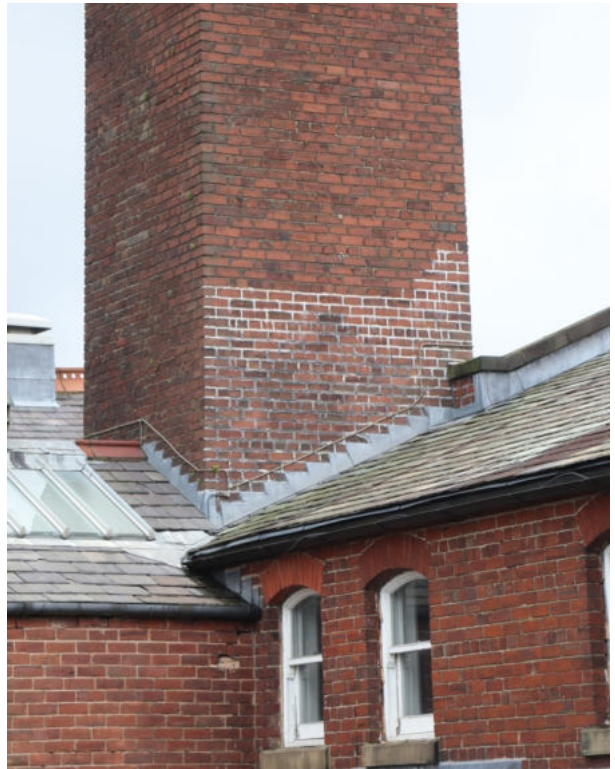
06 & 07 (Area D). Damage to finishes from water ingress above lift shaft (lift 1) and recent repointing works, which have made an improvement to the water ingress.
