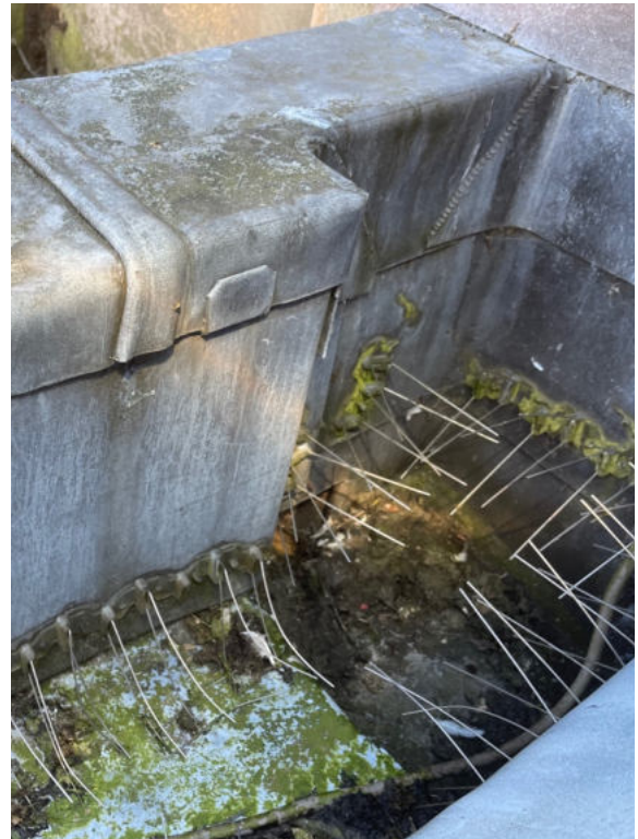
02 Area A (Note, Area B same but mirrored). Lead gutter discharges onto cornice, through channel cut into stone and lined in lead. Capacity is very limited and there is in effect no catch-pit or sump.
