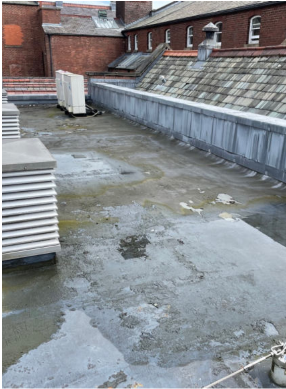
05 (Area F). Evidence of ponding to the flat roof, extensive coating failure and patching. Right, internal water ingress and damage to finishes.
