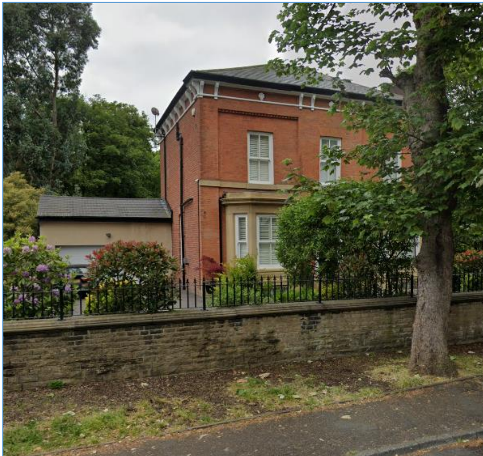
Figure 6: Garage at Dingle Bank.
