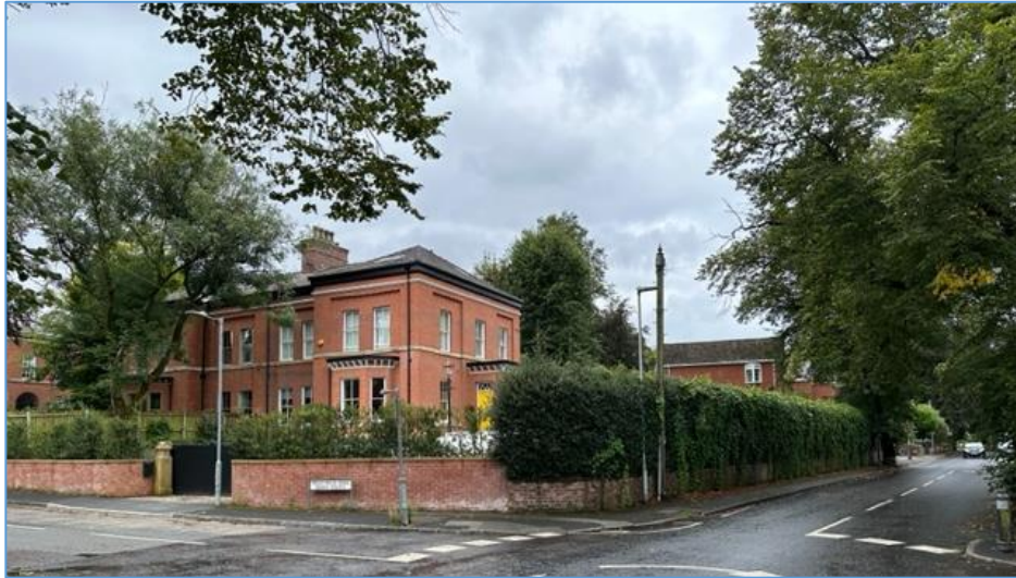
Figure 2: Hedging largely conceals the garage from view from St Ann's Road.
