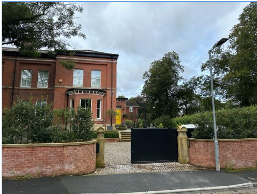
Figure 1: Image of the appeal site, viewed from the front.
