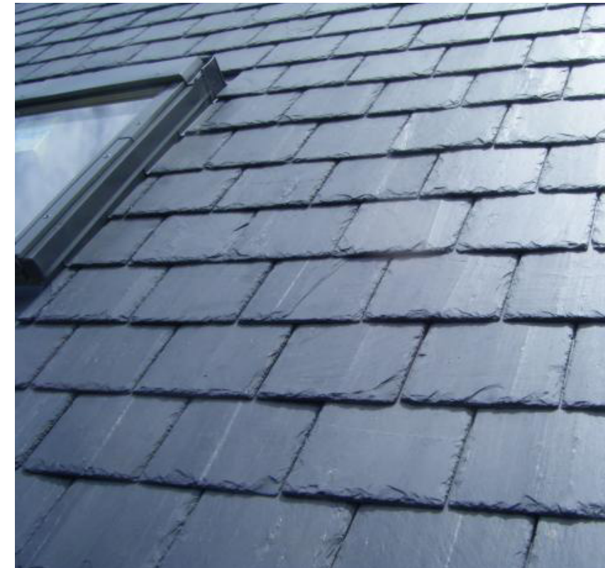
Fig 17 : Slate roofing with roof window
