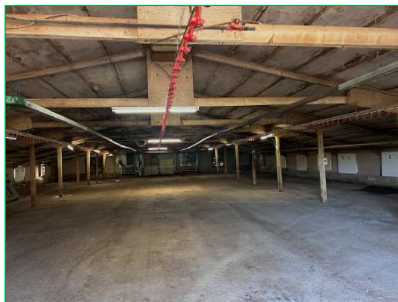
The internal structure of the agricultural building
