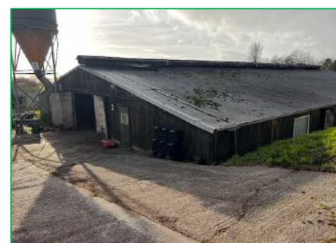
Developed land; sealed surface (agricultural building and adjacent hard standing)
